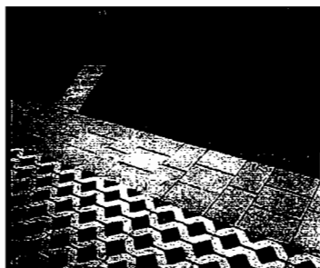
Permeable pavement allows water infiltration, reduces run-off
