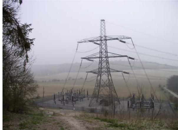
**Transition stations are used to connect lines and cables together**
