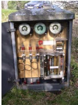
**Kiosk containing pressure gauges and fluid leak alarms**
