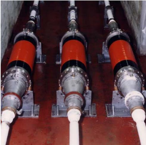
**Joints near completion in a joint bay, they will later be buried with soil up to street level**
