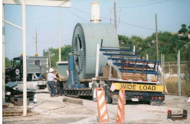
**Reel being prepared for cable pulling**
