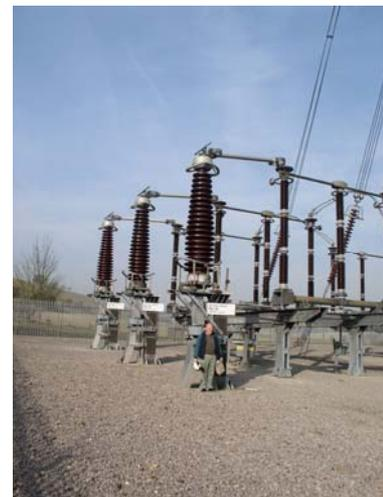
**Transition stations where cable terminations are connected to overhead lines**
