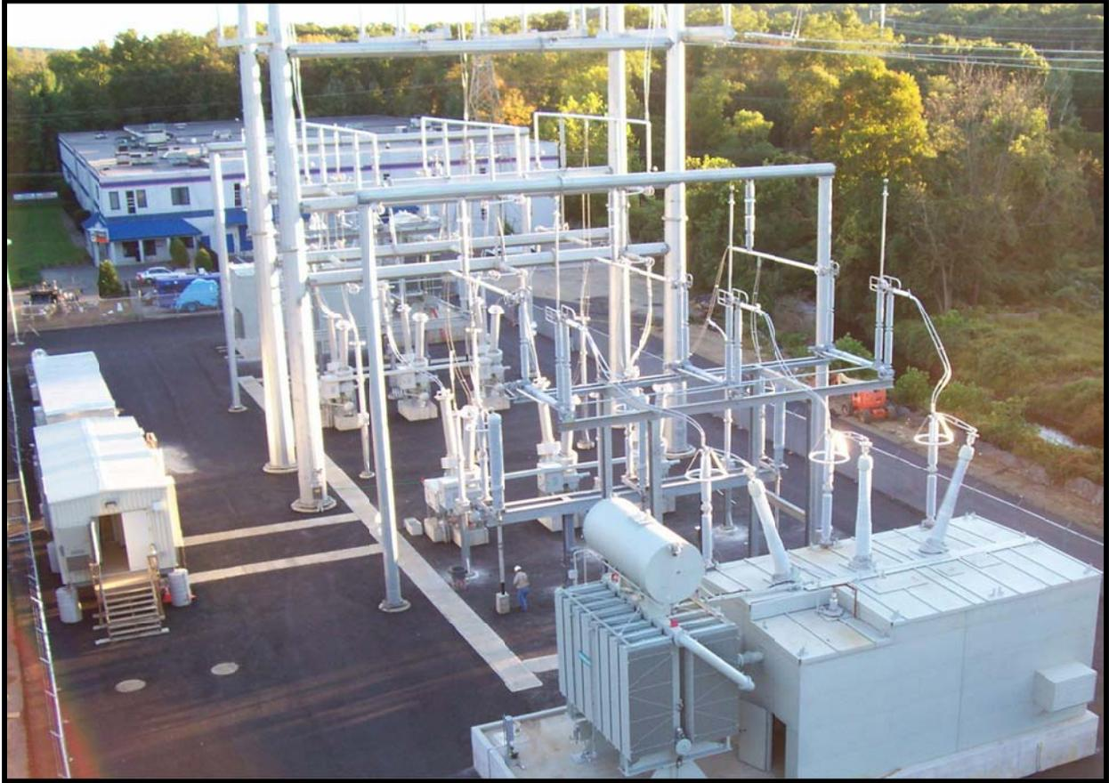
**Figure 15A-3: 345-kV Line Transition Station with no Shunt Reactors**
