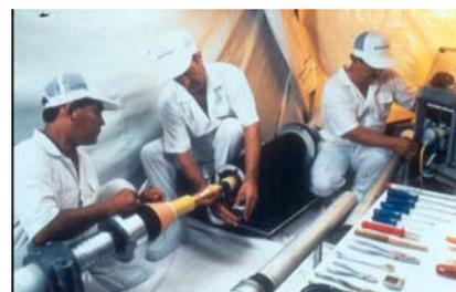
**Connecting XLPE cables together in an ultra-clean environment within a buried joint bay**
