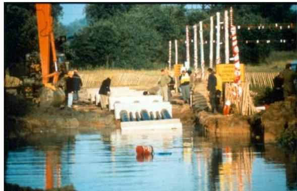
**Installation of ducts to house the cables that will cross the river**
