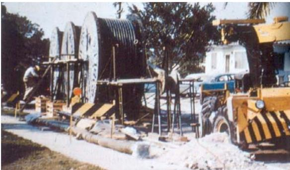
**Three reels of cable are parked in the street ready to be pulled into a steel pipe**
