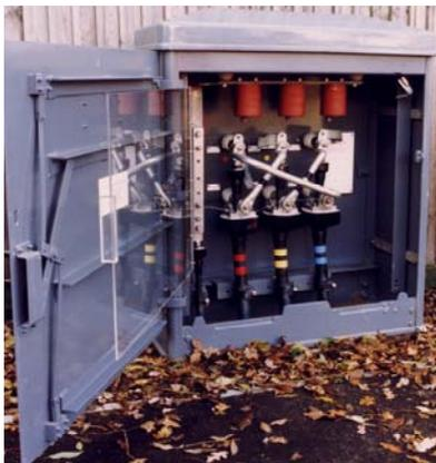
**A kiosk used to make electrical connections to ground**
