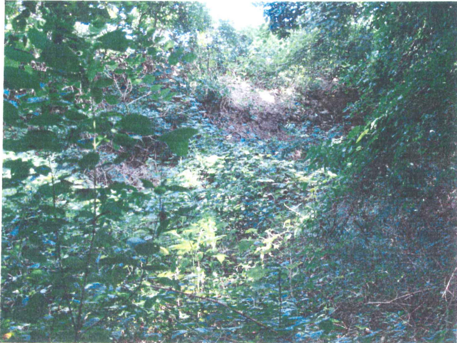
Photo 3 of 3: Riprap slope supporting former cinema parking in background (near W-4).
