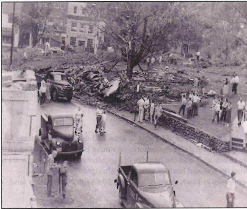
Cleanup after the 1938 Hurricane.
