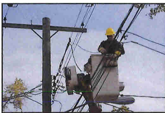
Cable is provided by Comcast, while wireline telephone is provided by Frontier
