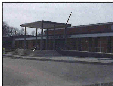
East Hampton High School During Construction
