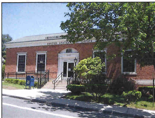
The East Hampton Post Office in the Village Center.
