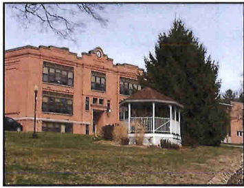
Center School in the Village Center houses the water system which supplies water to the center.
