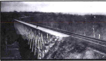
The Rapallo Viaduct in East Hampton spans Flat Brook on the Airline Railroad. Named for a director of the railroad, it is 1,380 feet long and 60 feet high. It was built out of iron in 1873, and later filled in when trains became heavier.
