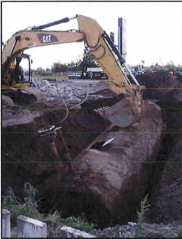
Removing Underground Storage Tanks is essential to protecting groundwater resources.
