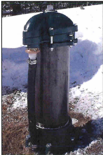
A typical water supply wellhead consists of a cap and seal, as well as an air vent. East Hampton relies primarily on private wells on individual properties.
