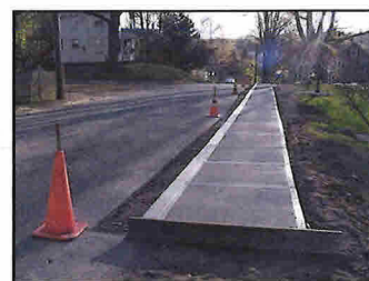
Sidewalk installation on Barton Hill
