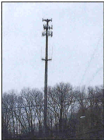
Cell towers such as this one near the Public Works Department provide for wireless services.
