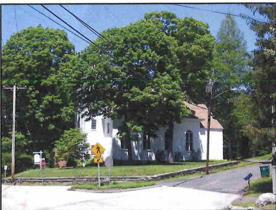
The Middle Haddam Episcopal Church seen here is located in the Middle Haddam National Historic District.
