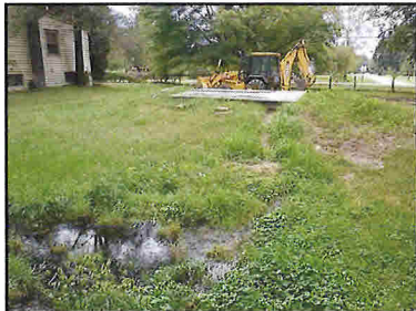
Failing Septic System
