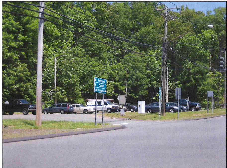
East Hampton Park & Ride Facility at the Intersection of Routes 16 & 66
