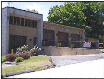
East Hampton Fire Headquarters
