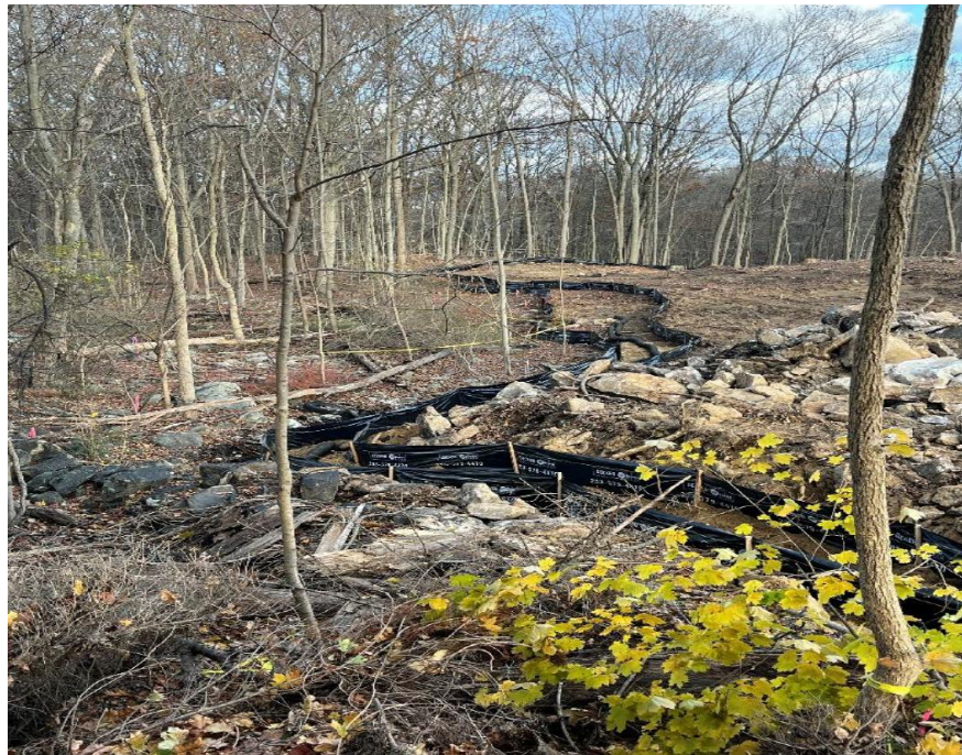
Photo 3: Redundant erosion and sediment control barrier between disturbed areas and adjacent wetlands.
