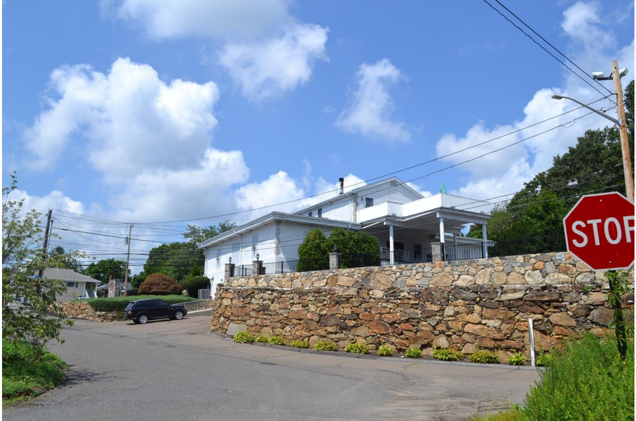
Photograph 12: View looking northwest away from the Project Area from Kaechele Place. 8/8/2019.
