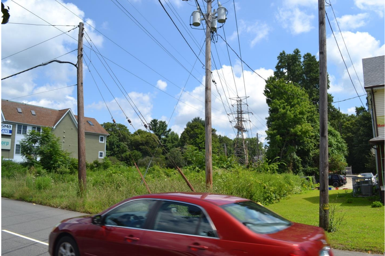
Photograph 26: View looking northeast at the Project Area from Main Street. 8/8/2019.
