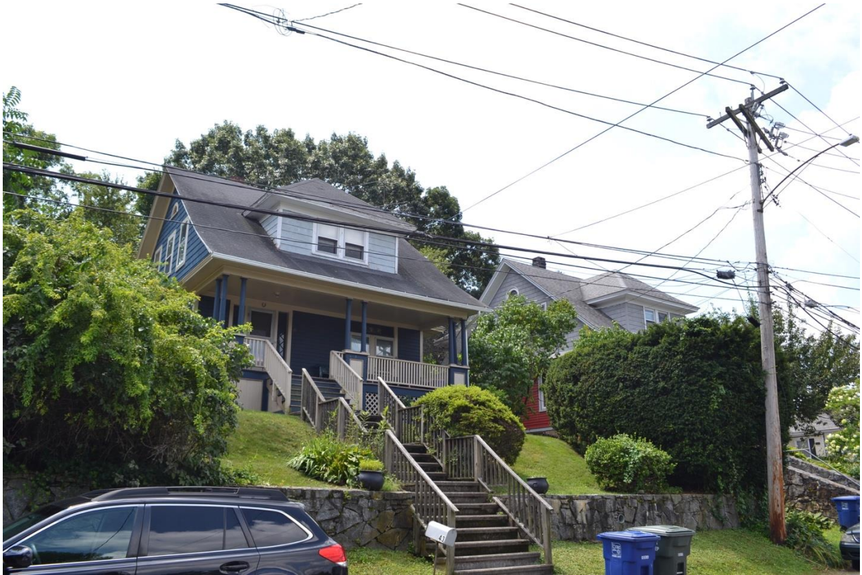
Photograph 19: View looking southwest away from the Project Area from Hillview Street. 8/8/2019.
