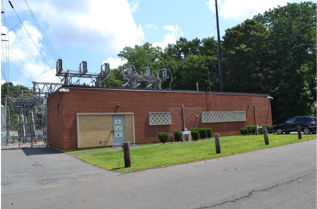
Photograph 6: View looking southeast at the Project Area from Kaechele Place. 8/8/2019.
