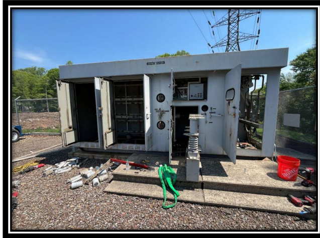
Photo 1: Capacitor bank and enclosure removals, typical.
