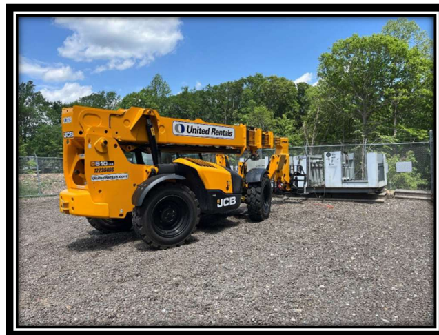
Photo 2: Removal of enclosure, typical.
