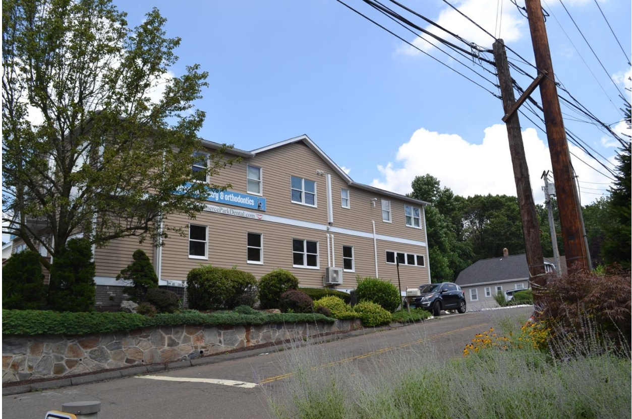
Photograph 23: View looking northeast towards the Project Area from the intersection of Hillview and Main Streets. 8/8/2019.
