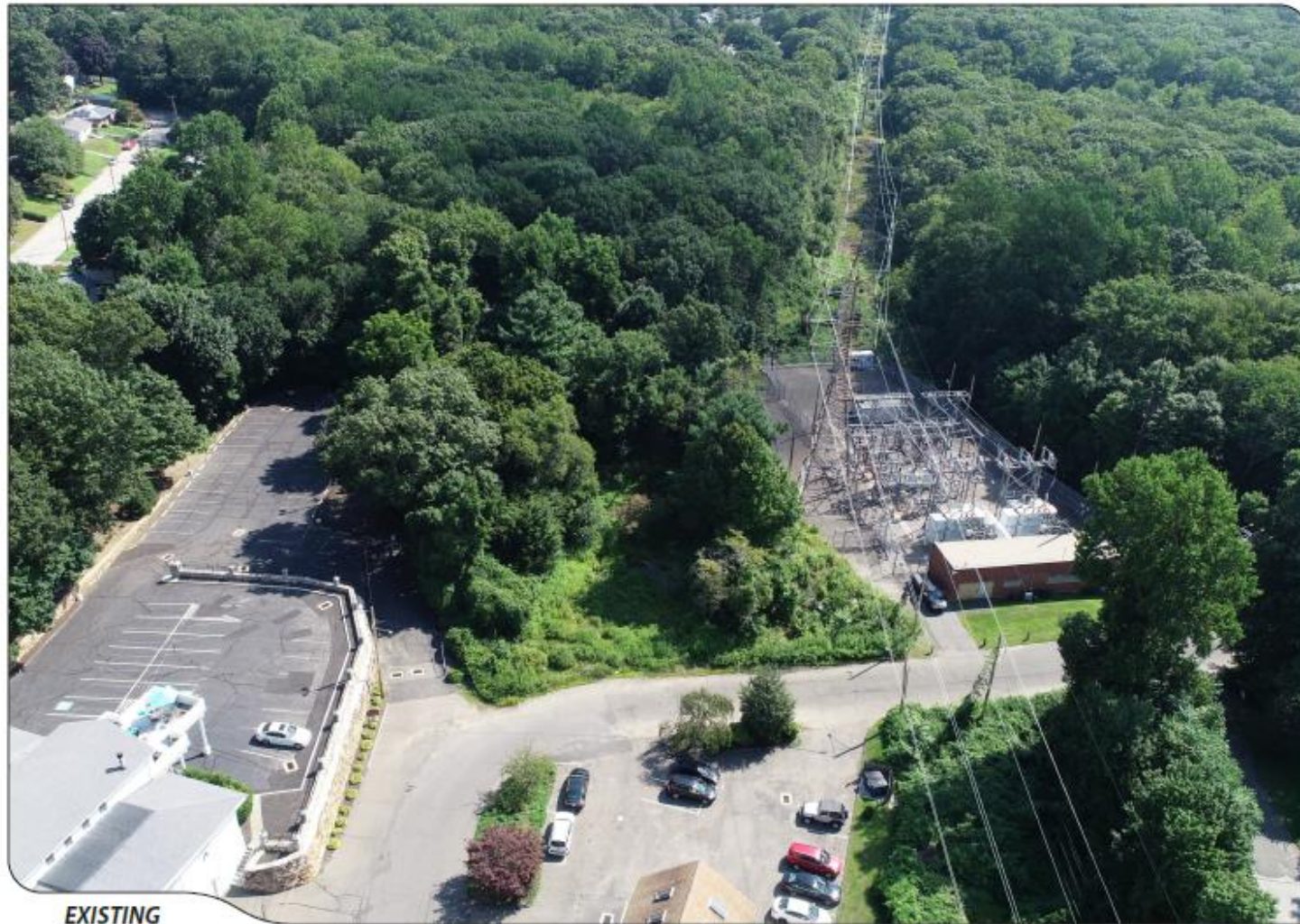
Figure 4-4: Representative View of Existing Old Town Substation, UI Property, Eversource ROW, and Immediate Vicinity (View to the East)
