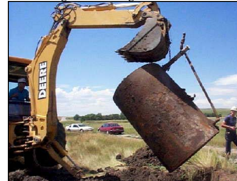
Underground Storage Tank Removal
