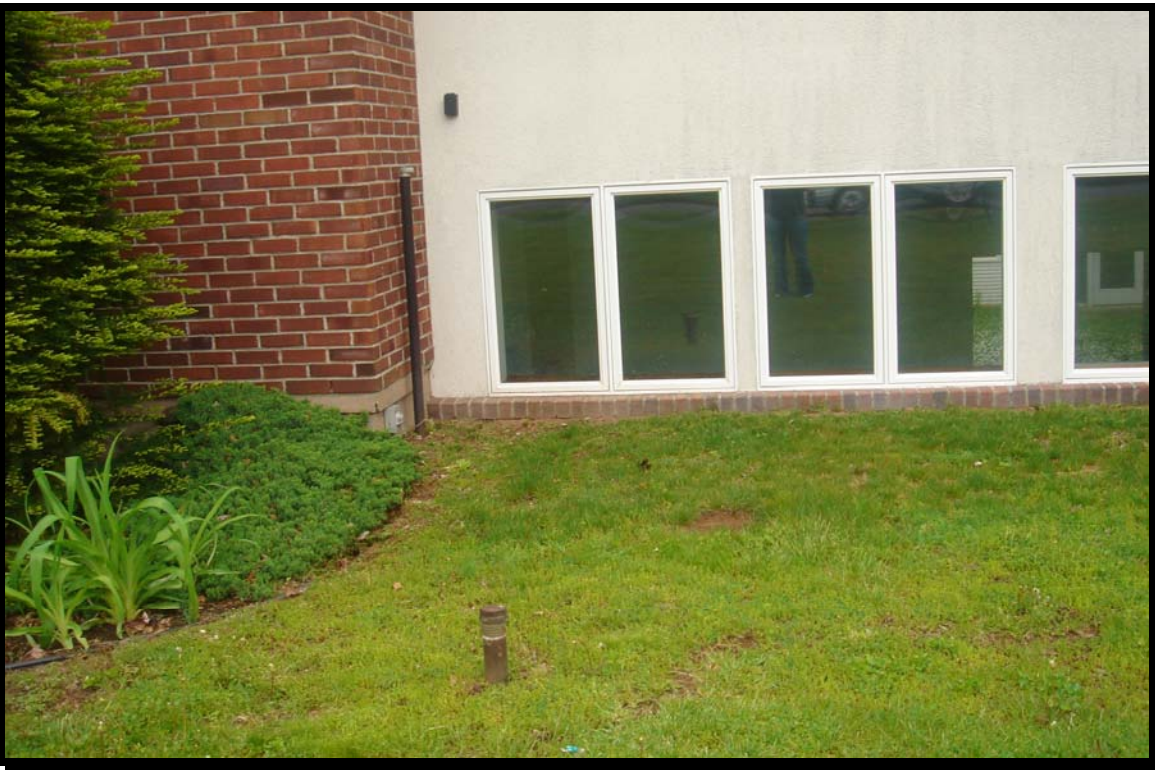
Vent and fills pipes of UST located east of southern portion of church building.
