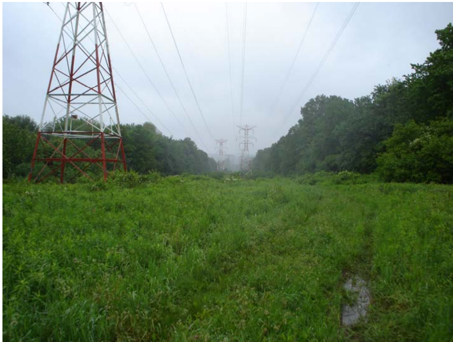
View of Existing CL&P Transmission Lines Intersecting Substation Parcel Looking North
