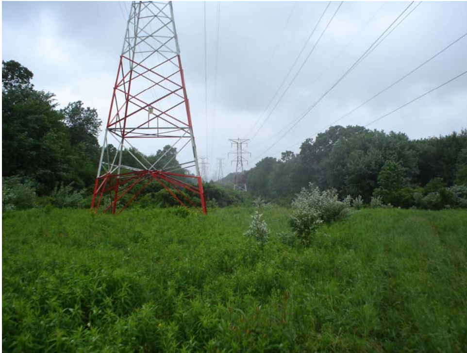
View of Existing CL&P Transmission Lines Looking Further North
