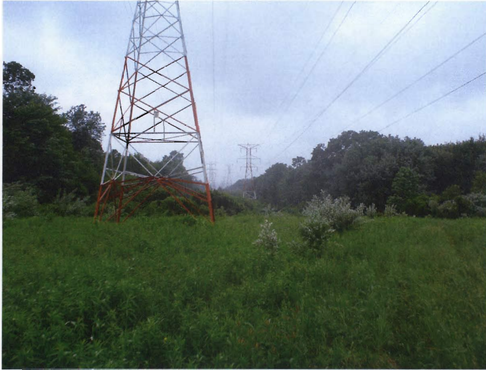
View of Existing CL&P Transmission Lines Looking Further North
