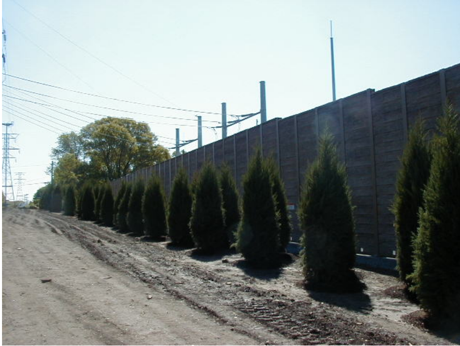
Figure A-1. Substation wall on north side of Trumbull substation.
