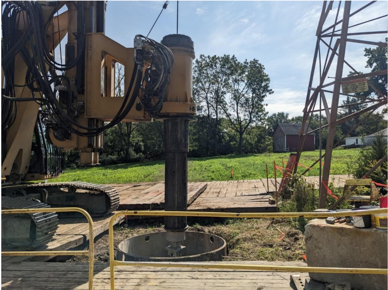
Photo 3: Drilling activities at STR 354.
