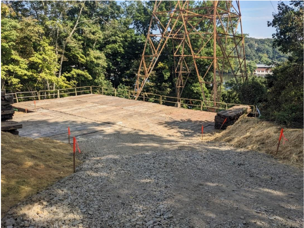
Photo 6: Completed installation of lower work pad at ST 359.
