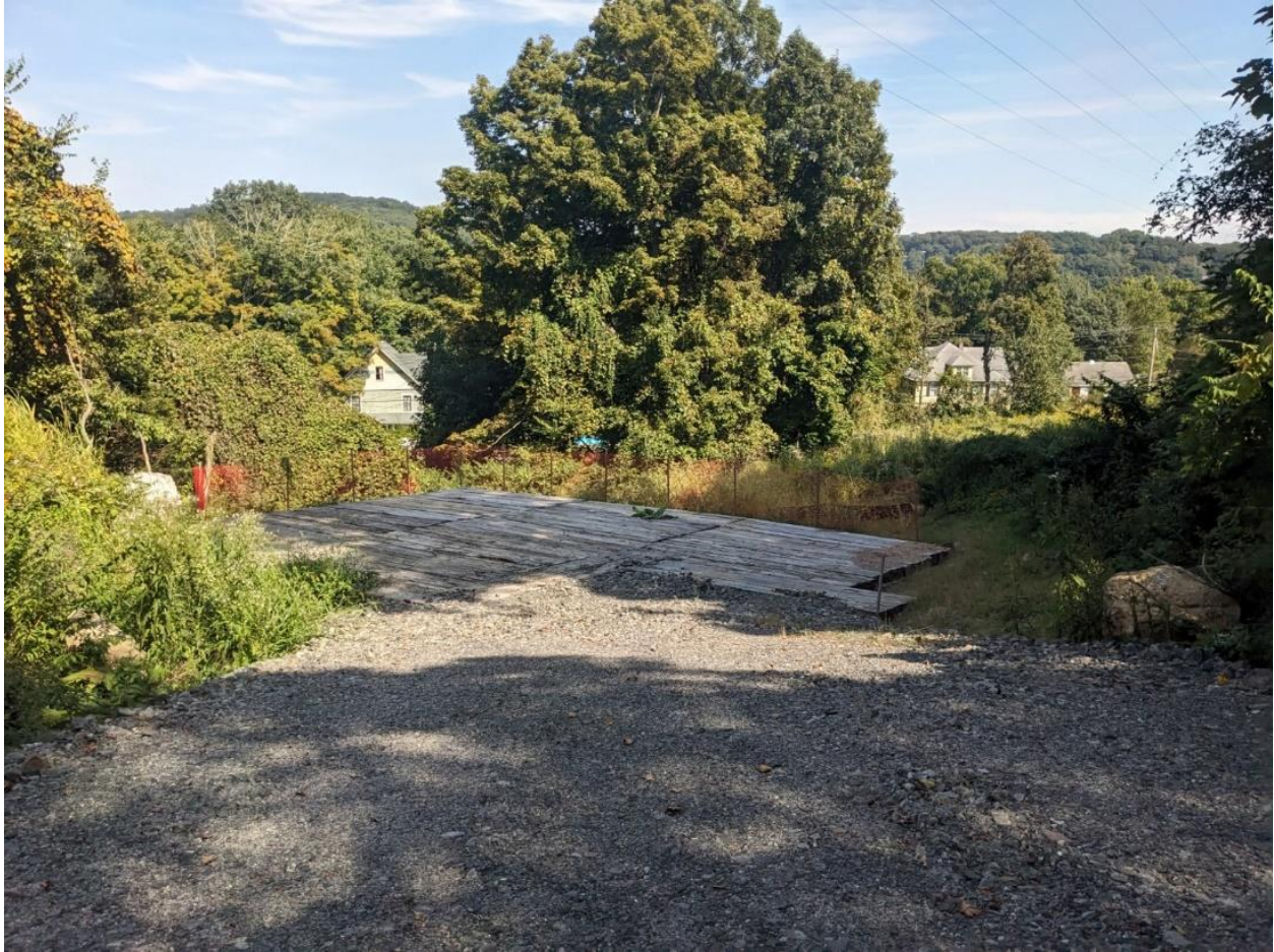
Photo 5: STR 358 work pad.
