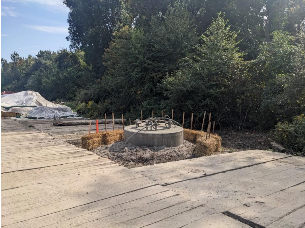
Photo 1: STR 350S concrete foundation installed.
