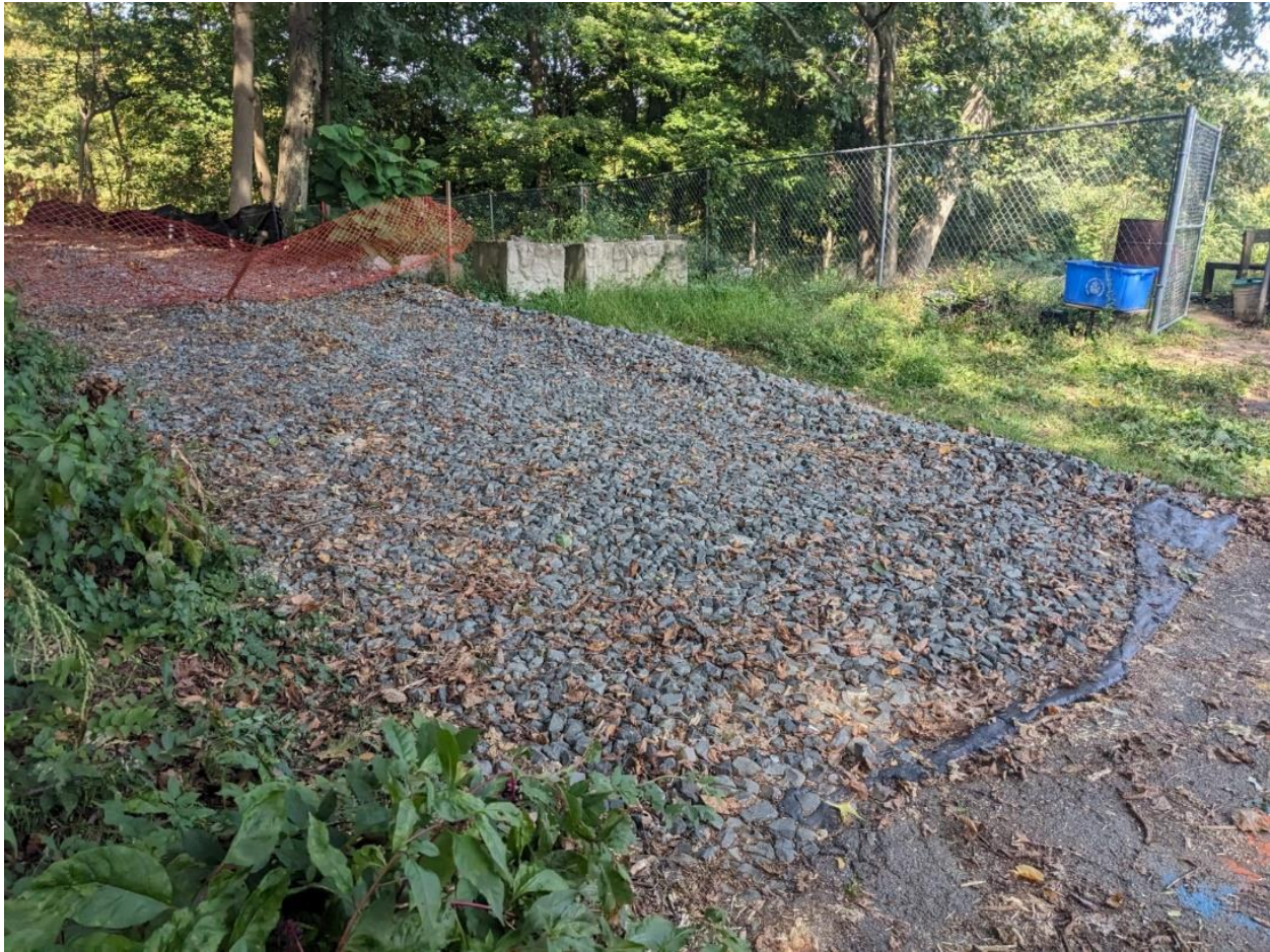
Photo 4: Construction entrance to STR 358 from Riverview Ave.
