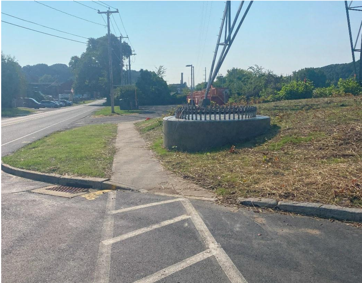
Photo 7: STR 360 concrete foundation installed.
