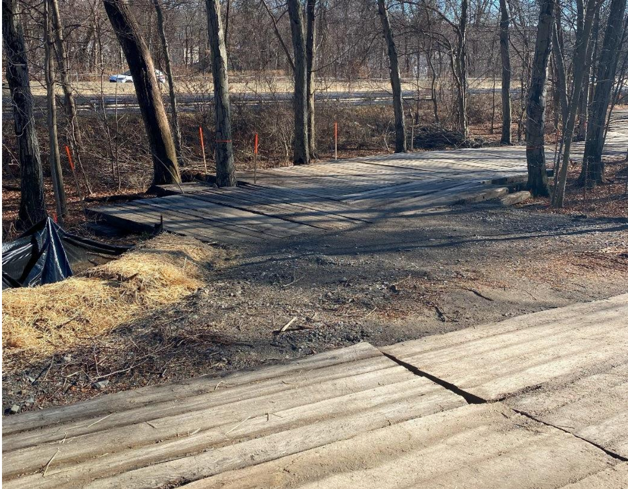
Photo 5: Temporary access at STR 14.
