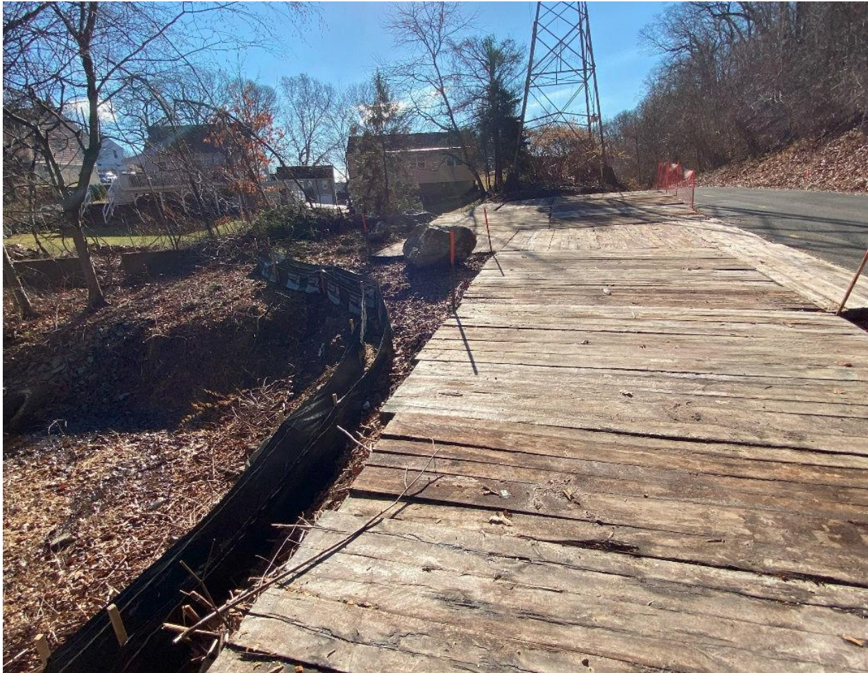
Photo 3: STR 6 work pad
