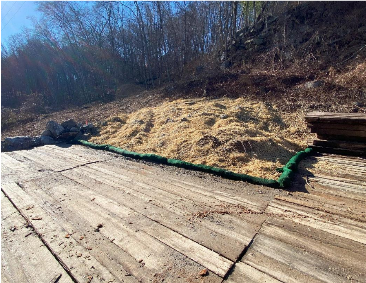
Photo 6: Stabilized soil at STR 14.
