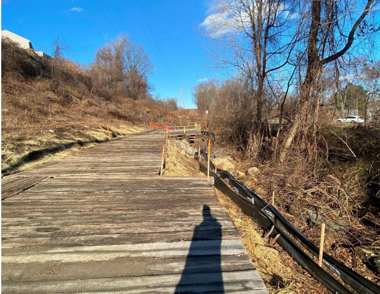
Photo 7: Construction pad at STR 14.
