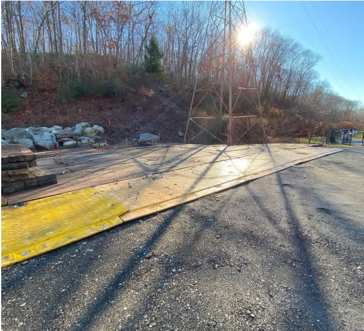
Photo 4: STR 8 matting installed
