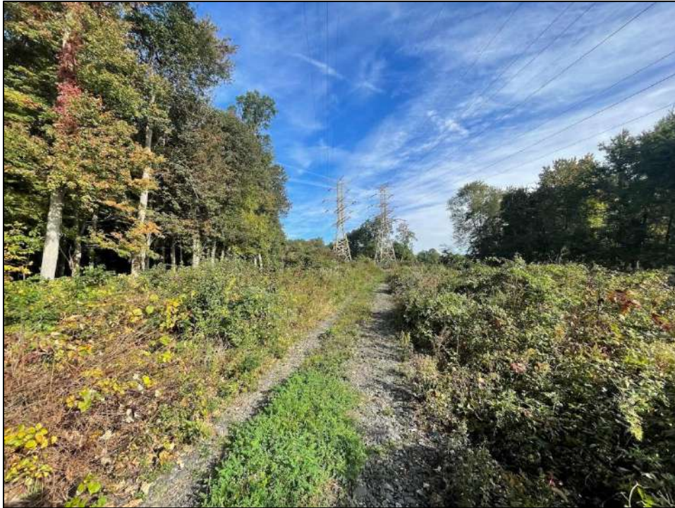
Photo 1. Overview photo showing proposed access road facing north towards Structure 350 (photo taken on October 12, 2021).
