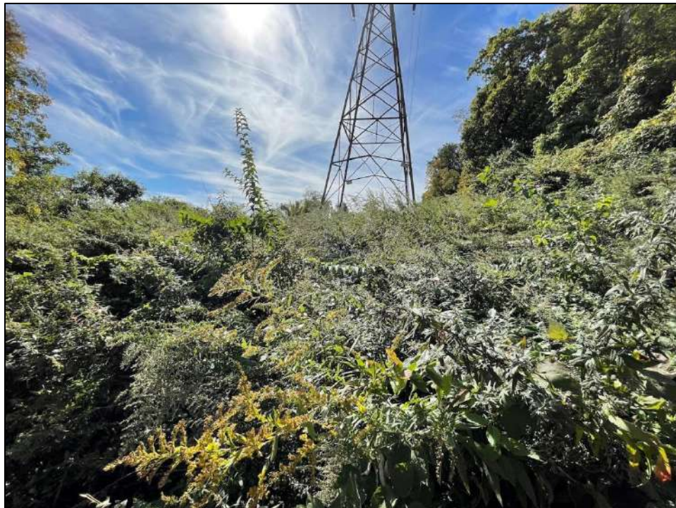
Photo 16. Overview photo of the project corridor facing south (photo taken on October 12, 2021).
