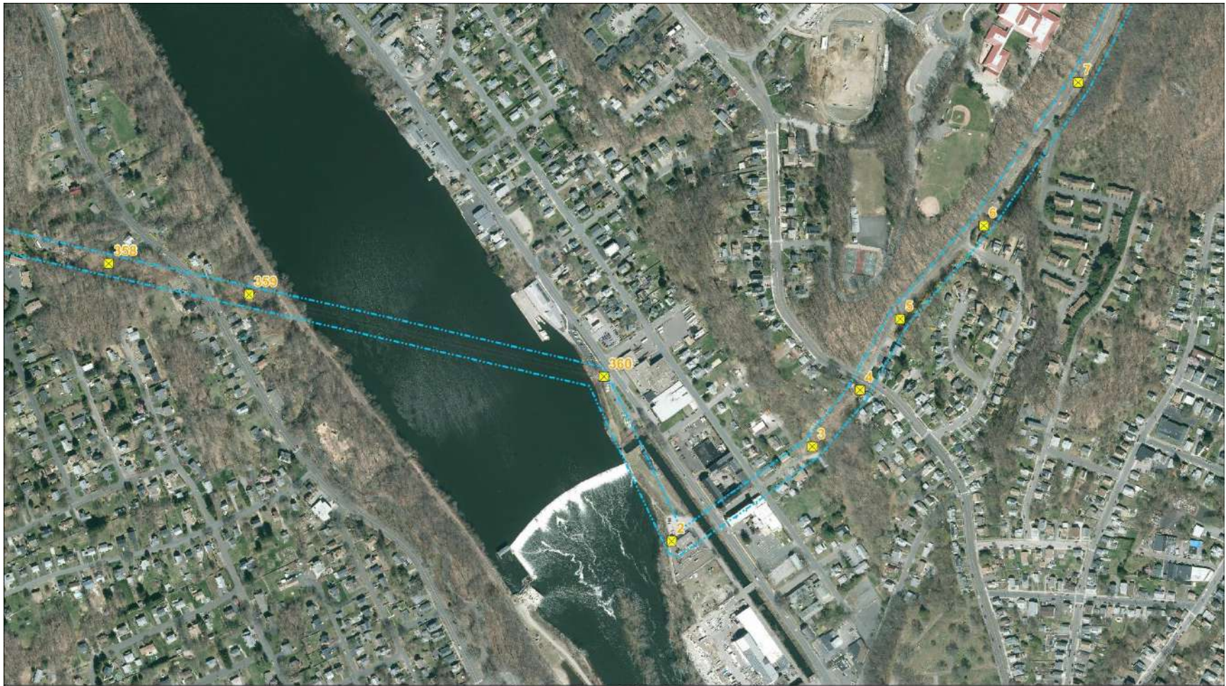
Derby Junction to Ansonia Substation, Connecticut
