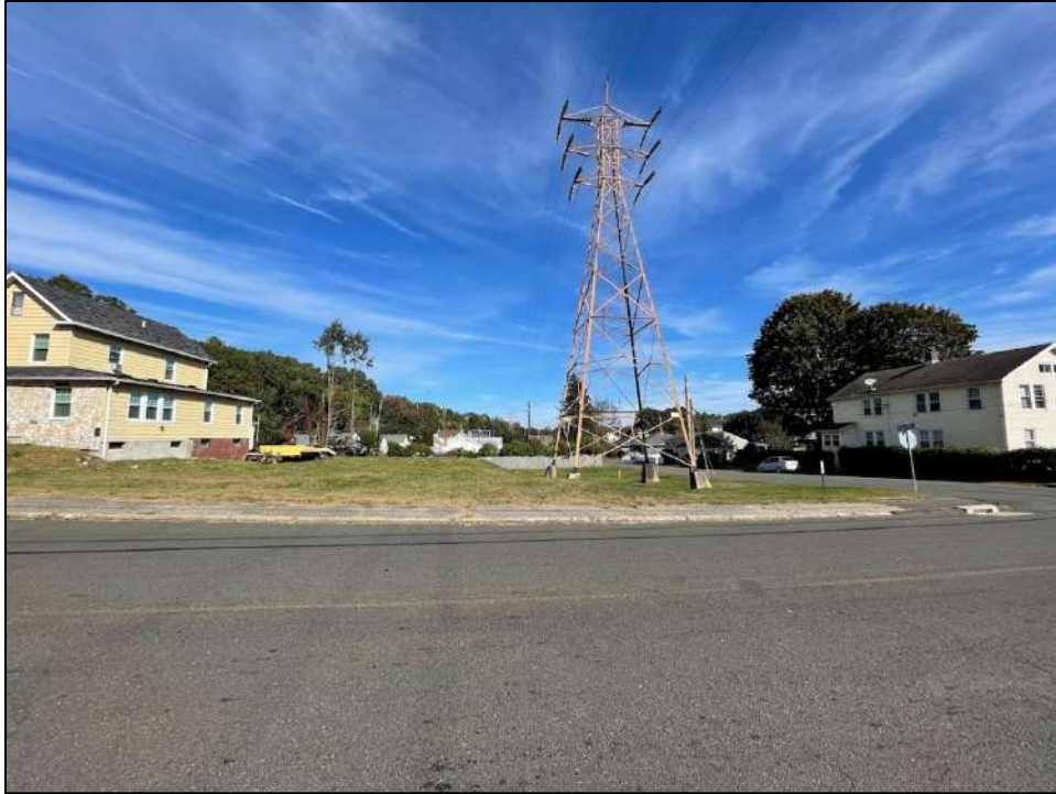
Photo 17. Overview photo of the project corridor facing north (photo taken on October 12, 2021).
