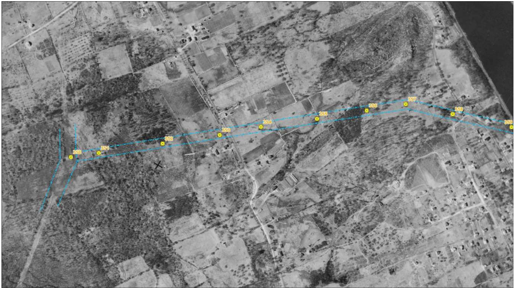
Derby Junction to Ansonia Substation, Connecticut
