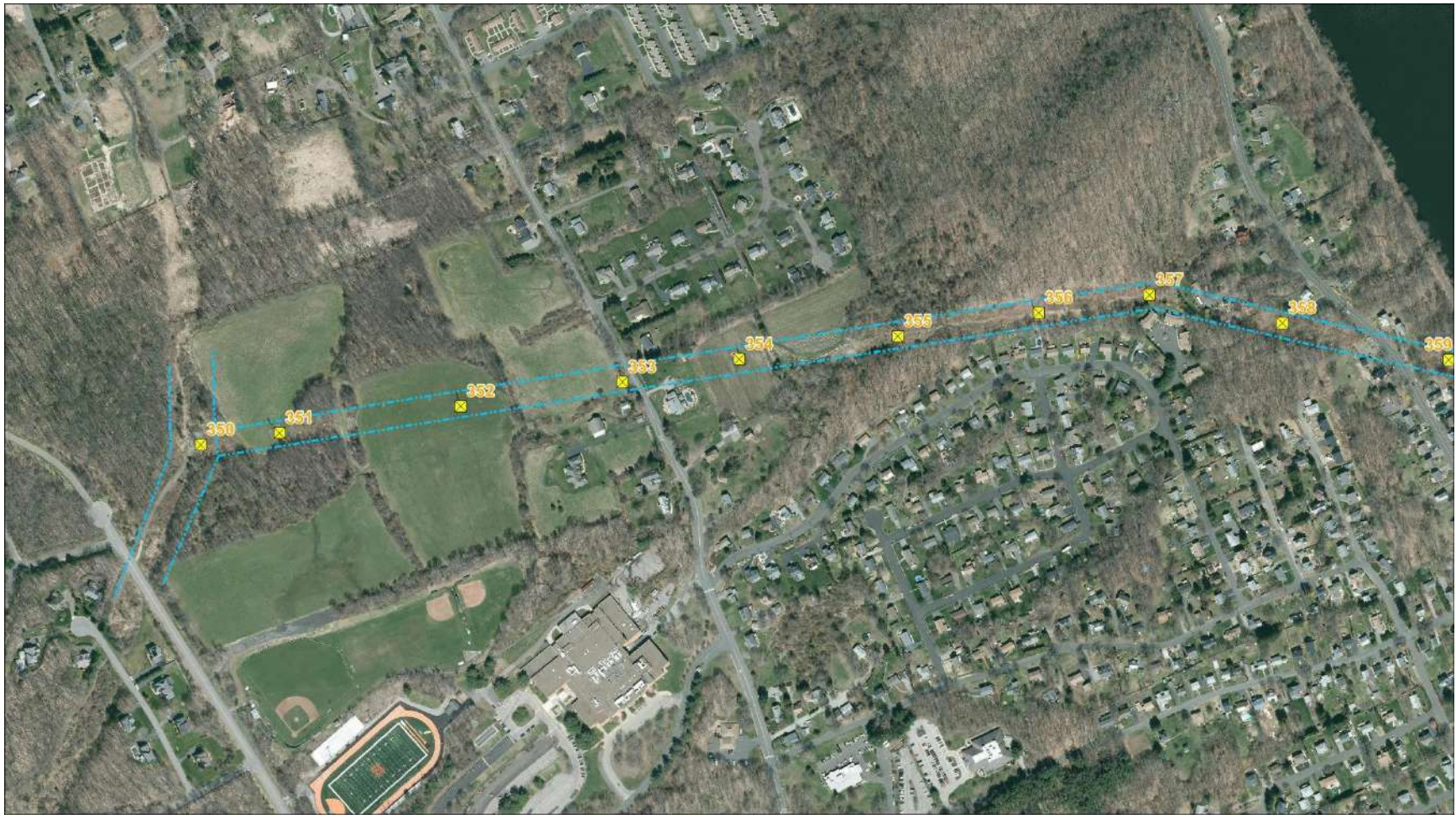
Derby Junction to Ansonia Substation, Connecticut
