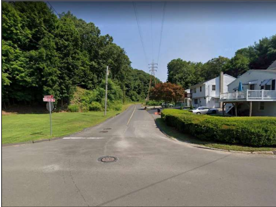
Photo 11. Overview photo of the project corridor facing north (photo taken on October 12, 2021).
