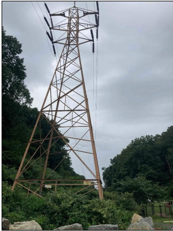
Photo 3: Overview of Ansonia-Derby T-line structure.
