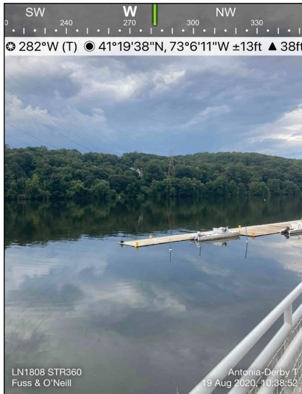
Photo 2: Overview of Ansonia-Derby T-line crossing Housatonic River.
