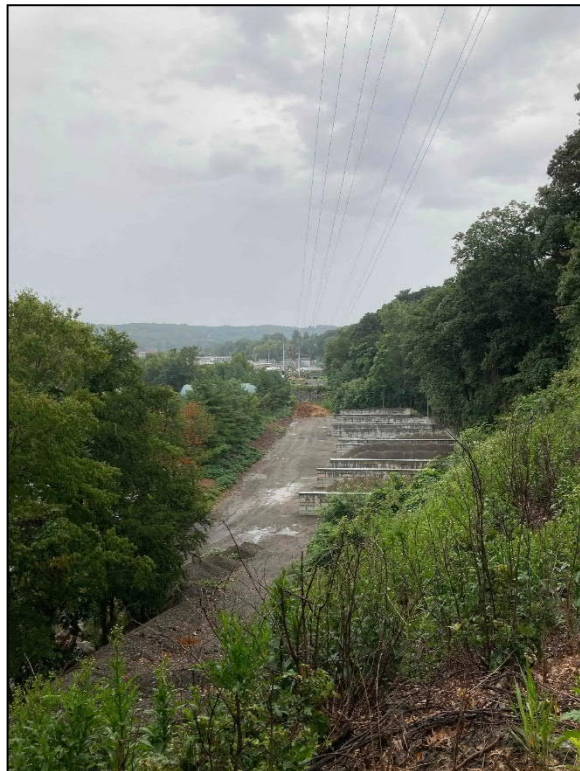
Photo 4: Overview of Ansonia-Derby T-line near Ansonia Substation.
