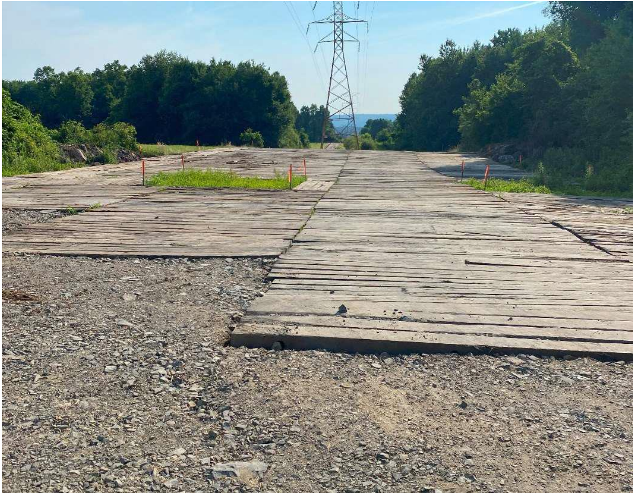
Photo 2: Temporary matting for Str. 350 & 351
