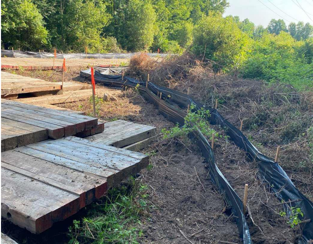
Photo 3: Double row sediment barrier along temporary matting at Str. 351
