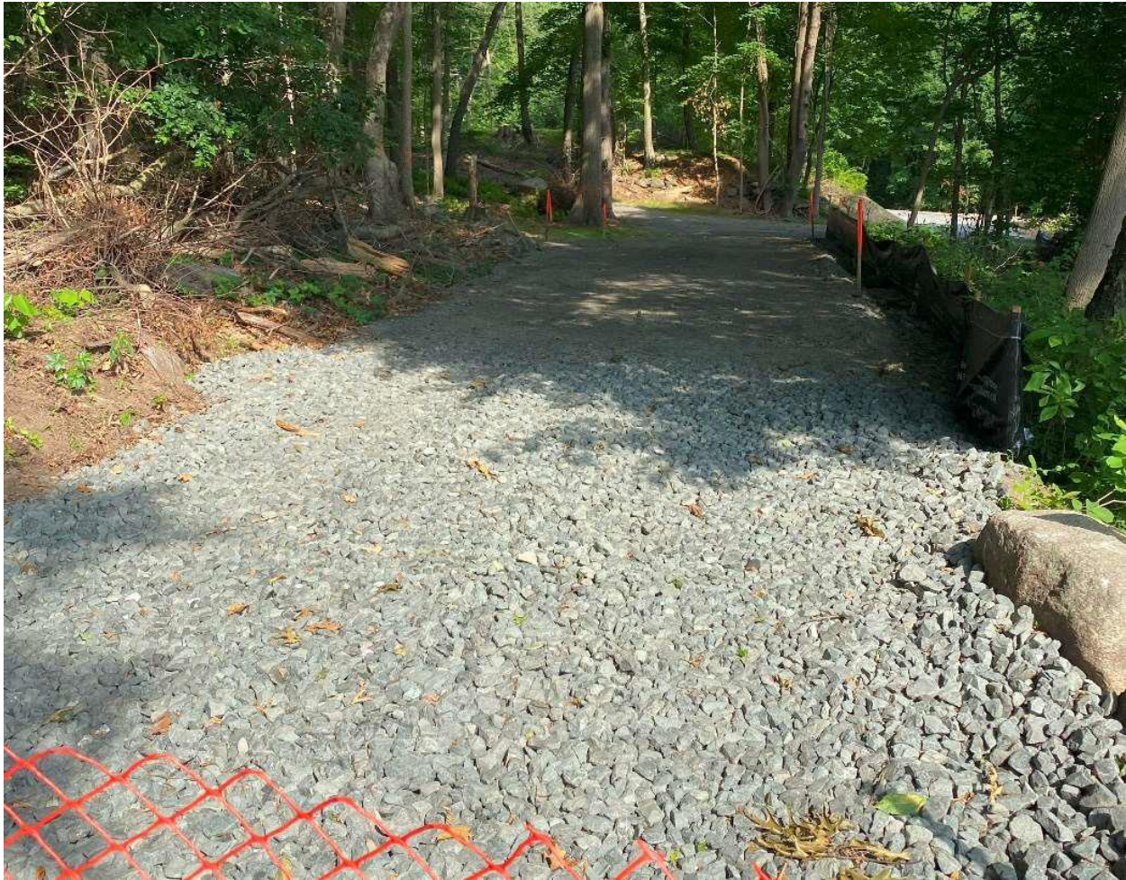
Photo 9: Rock construction entrance at Str. 358.
