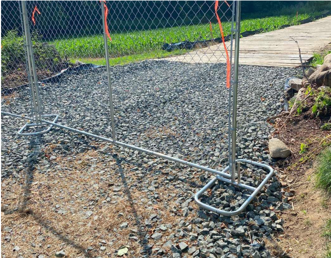
Photo 5: Rock construction entrance off Canterbury Ln.
