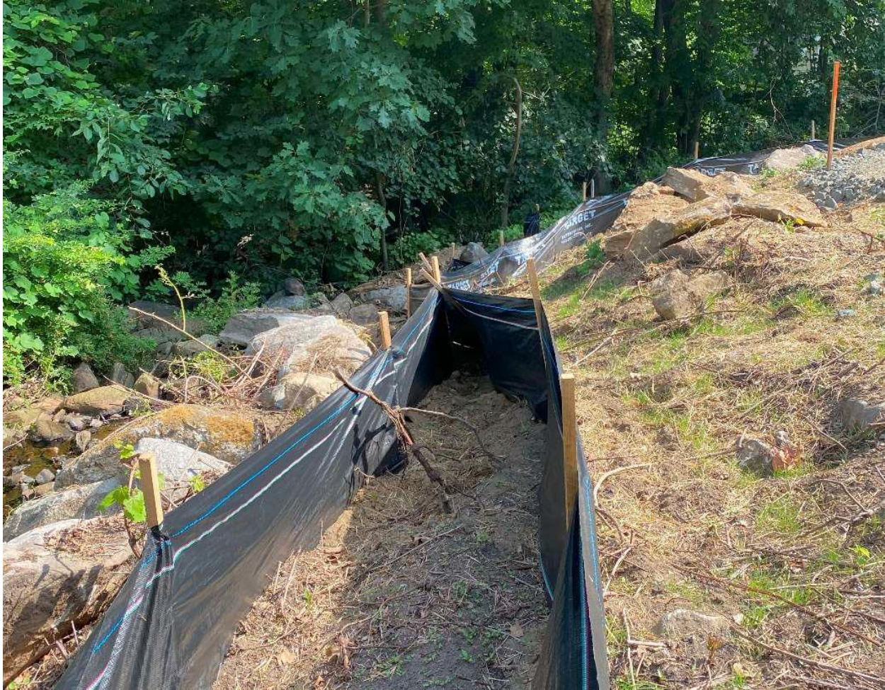
Photo 8: Double row sediment barrier along WC3 at western work pad at Str. 358.
