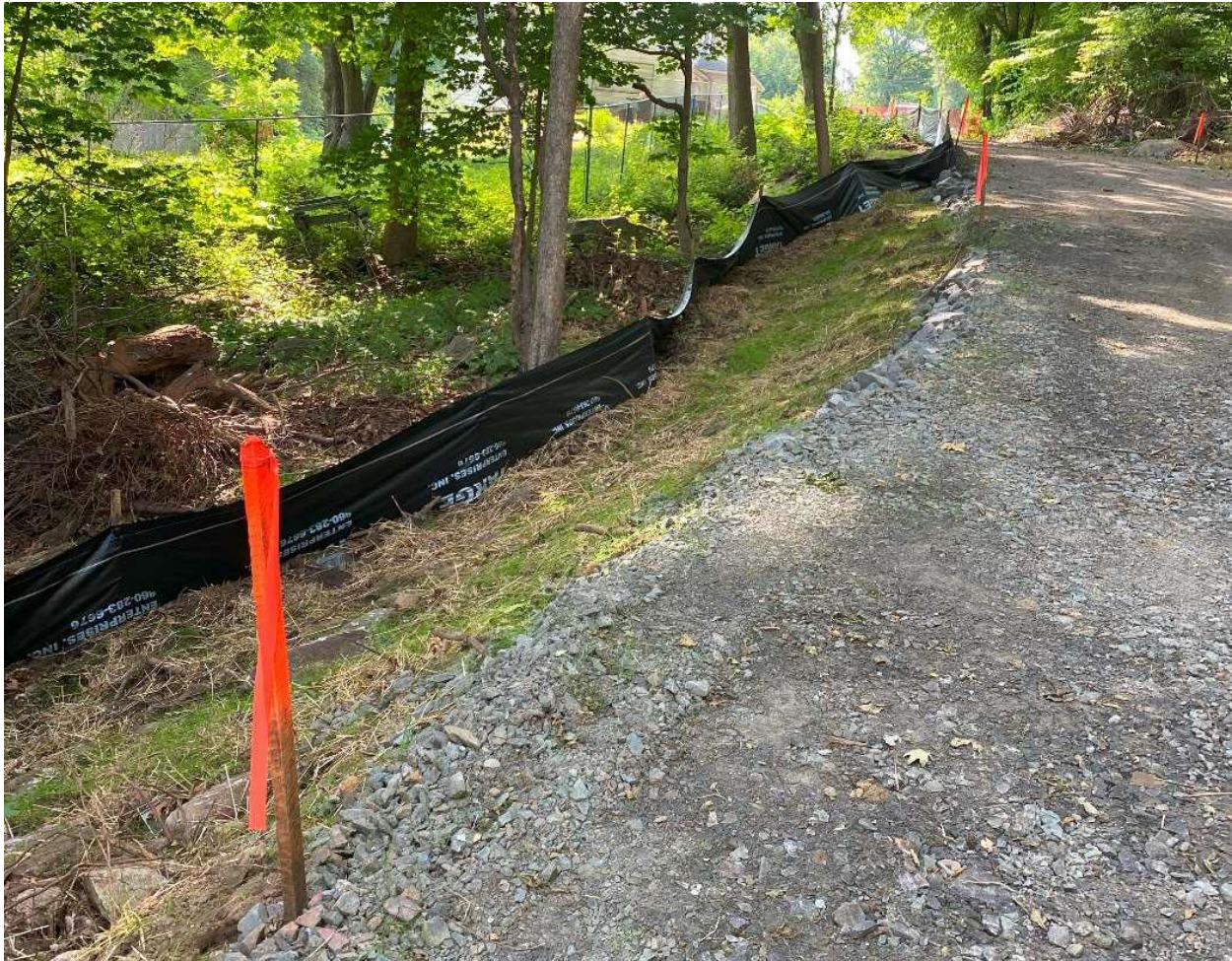
Photo 7: Sediment barrier along permanent access road at Str. 358
