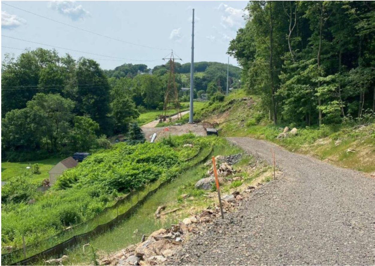
Photo 11: Permanent access road between STR 12 & 13
