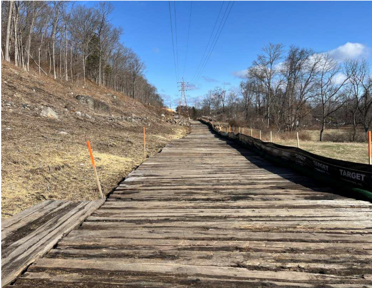
Photo 8: Temporary road construction looking towards Str. 12
