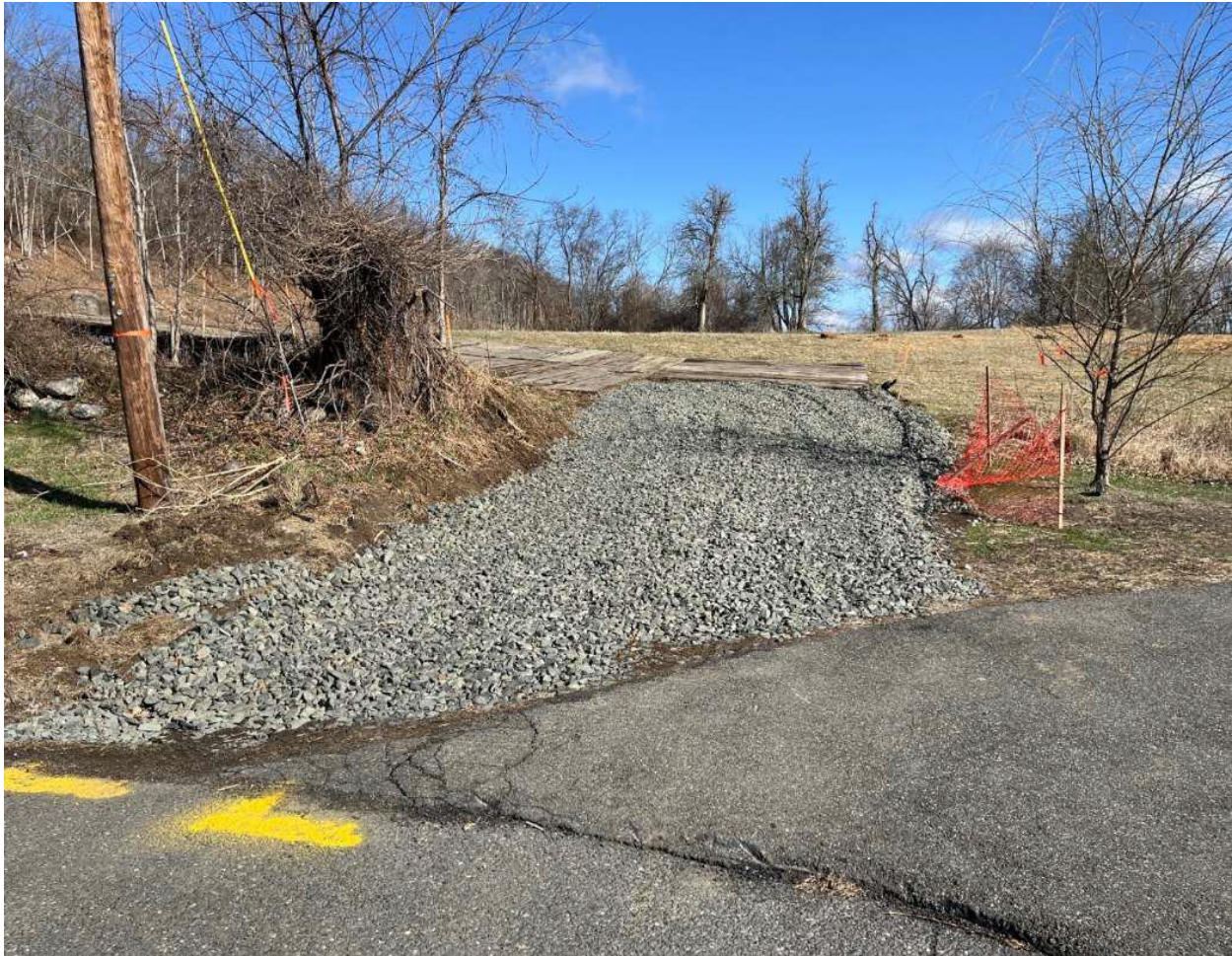
Photo 7: Rock construction entrance STR 11
