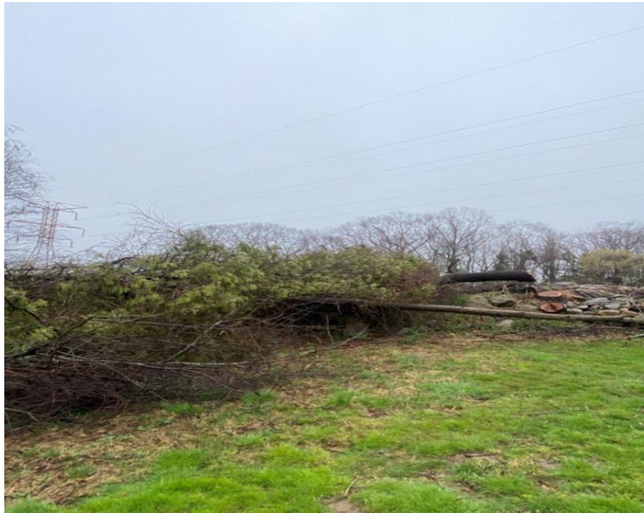
Photo 1: Clearing near Structure 355
