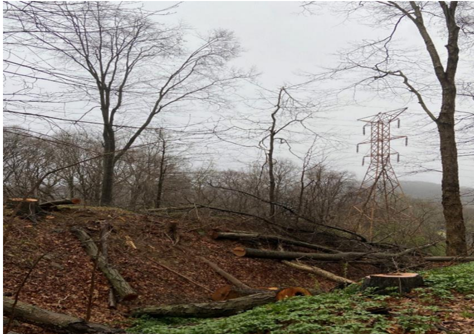
Photo 2: Clearing near Structure 358
