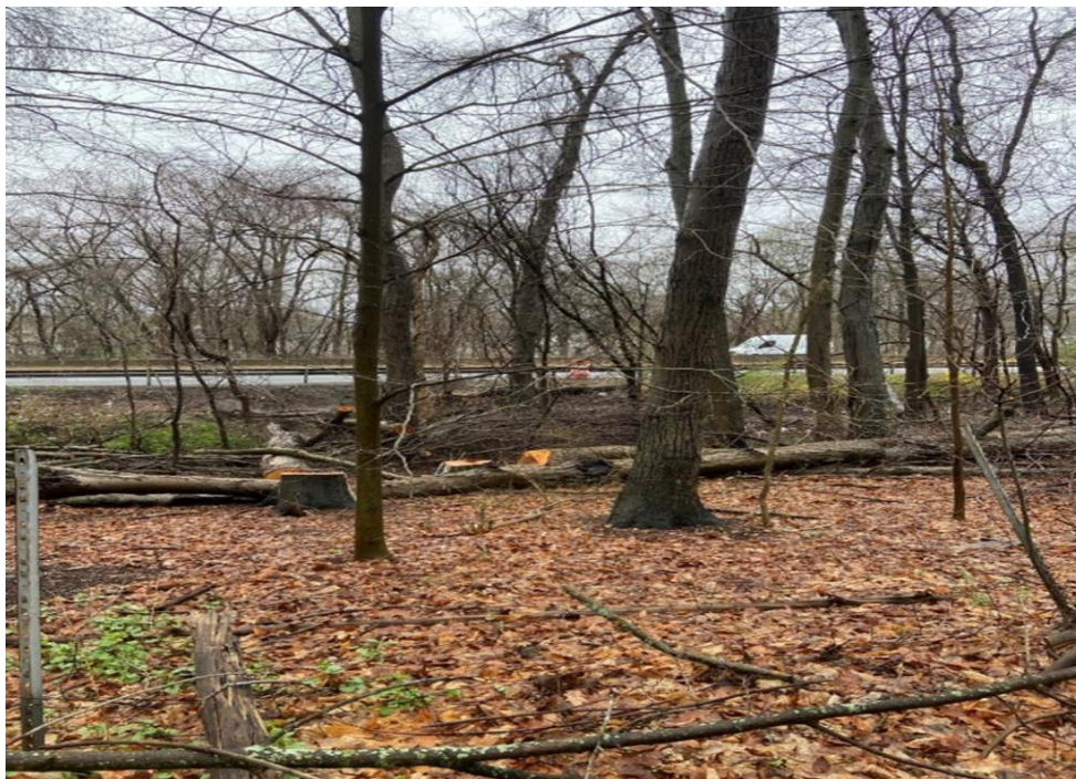
Photo 2: Clearing near Structure 14
