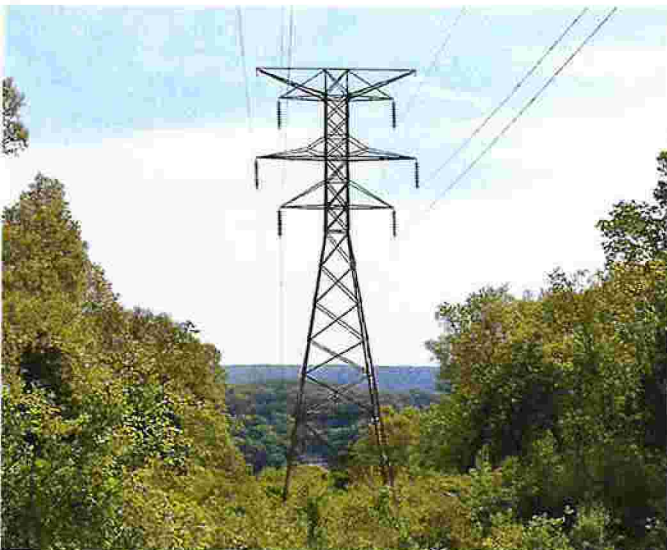
Typical existing lattice steel structure in Derby
