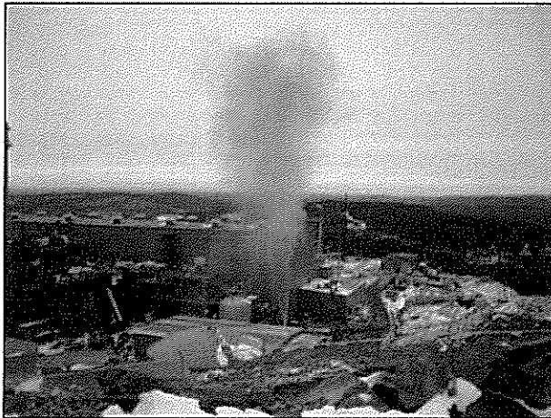
Figure 4-1 Iron Oxide and Debris Coming from Pipe
