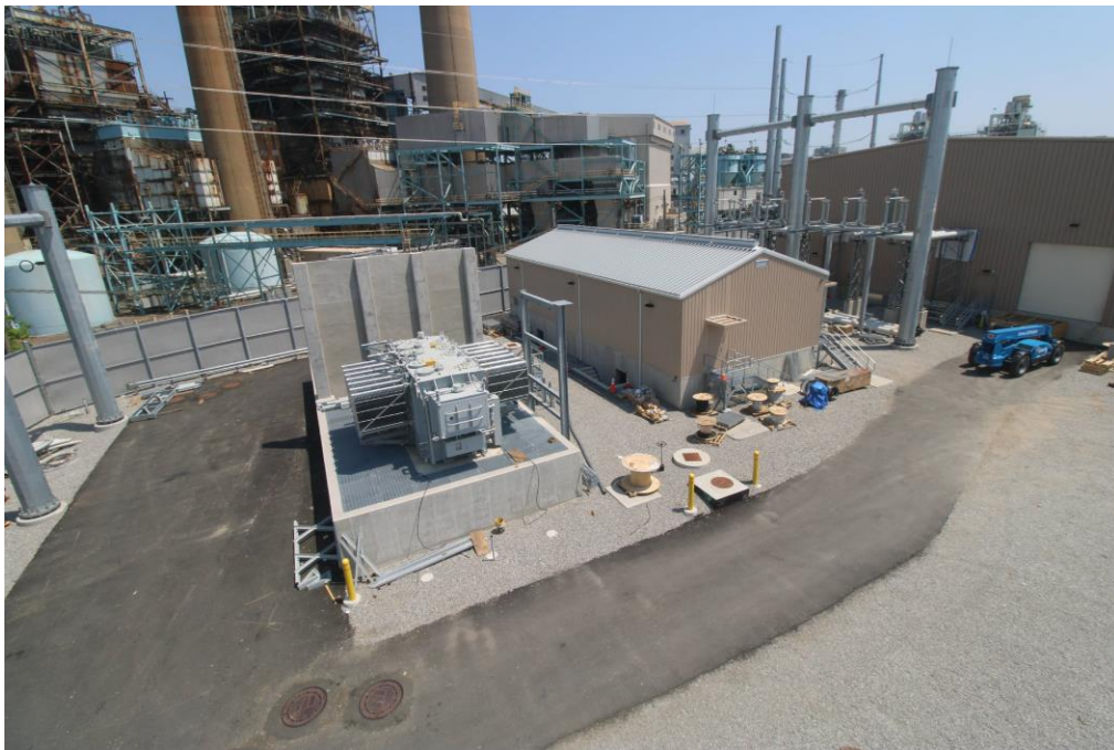
Photo 1: Broadview of project site with GIS/Control and PDC building exteriors completed.
