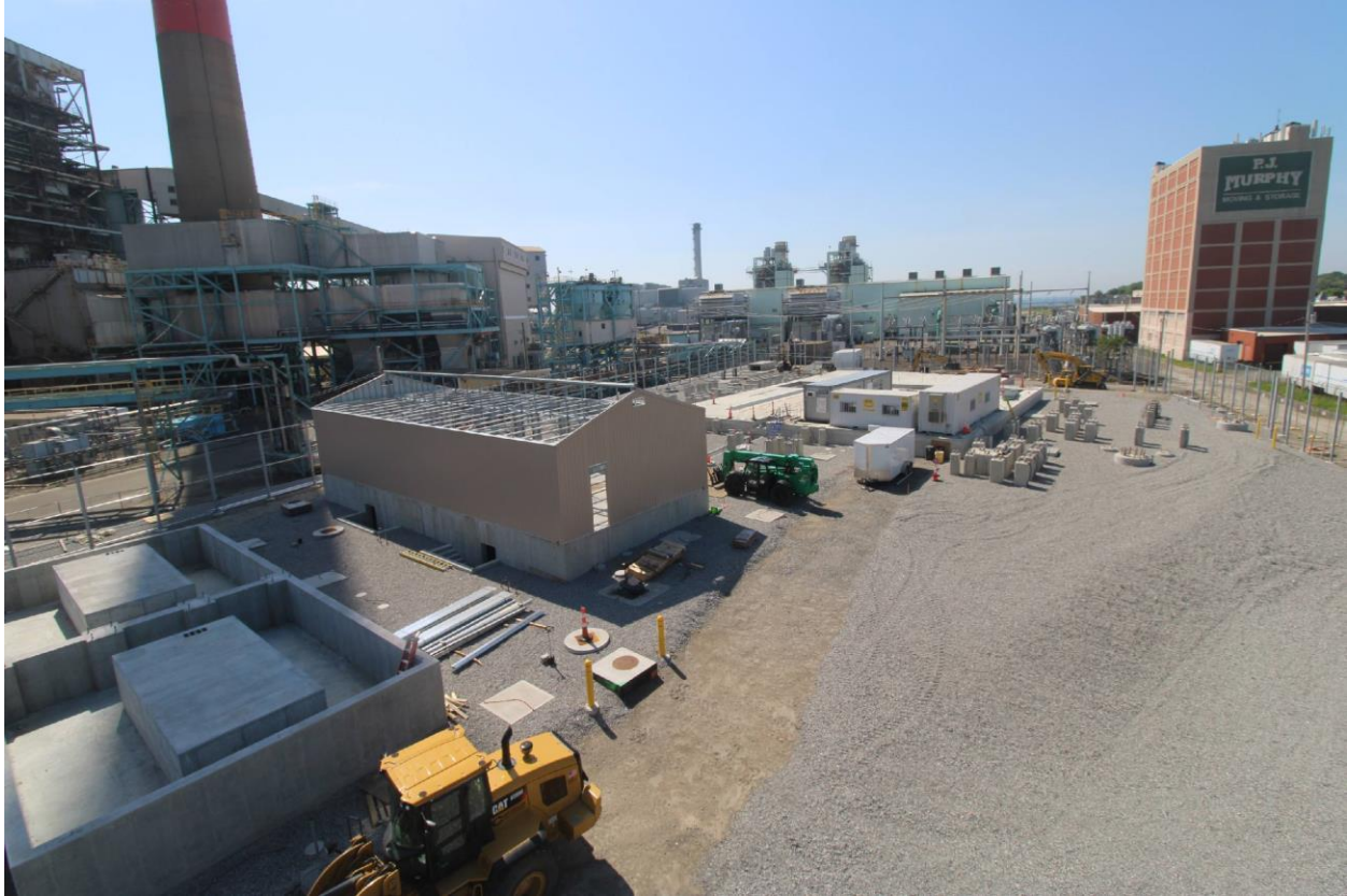
Photo 1: Broadview of project site with PDC Building being erected.
