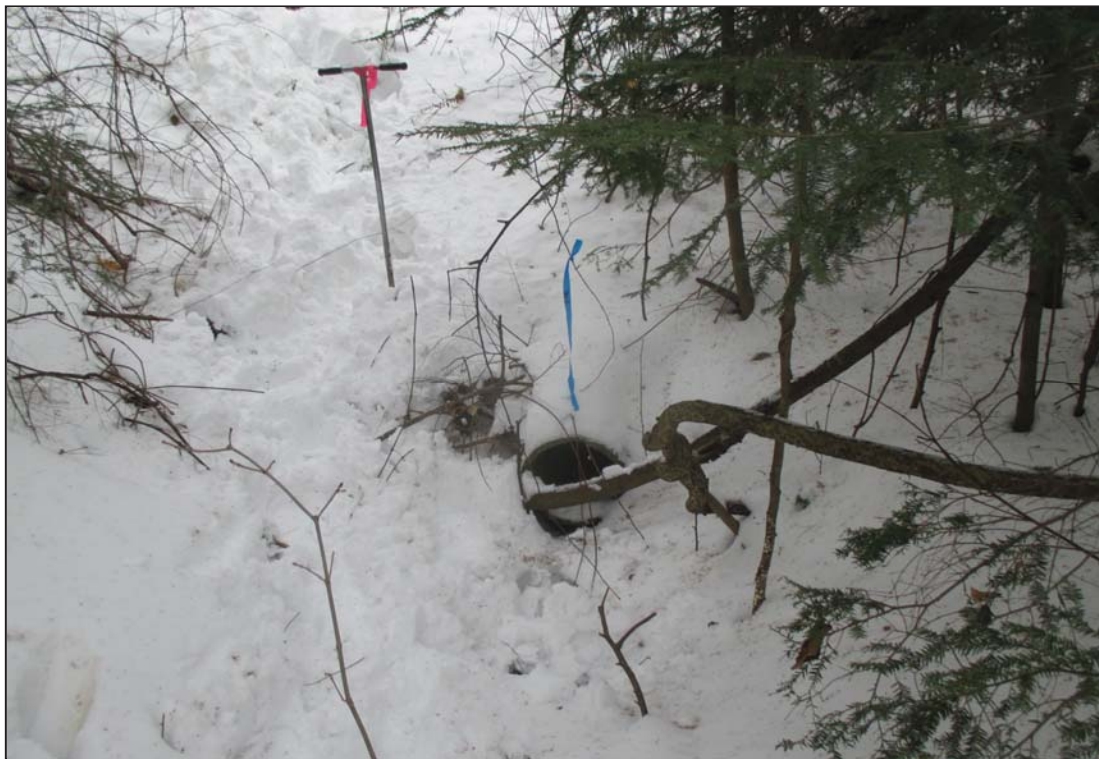
Photo 2: View of intermittent watercourse/12-inch RCP (JMM-IWC) (JMM photo taken 1/9/18); facing easterly
