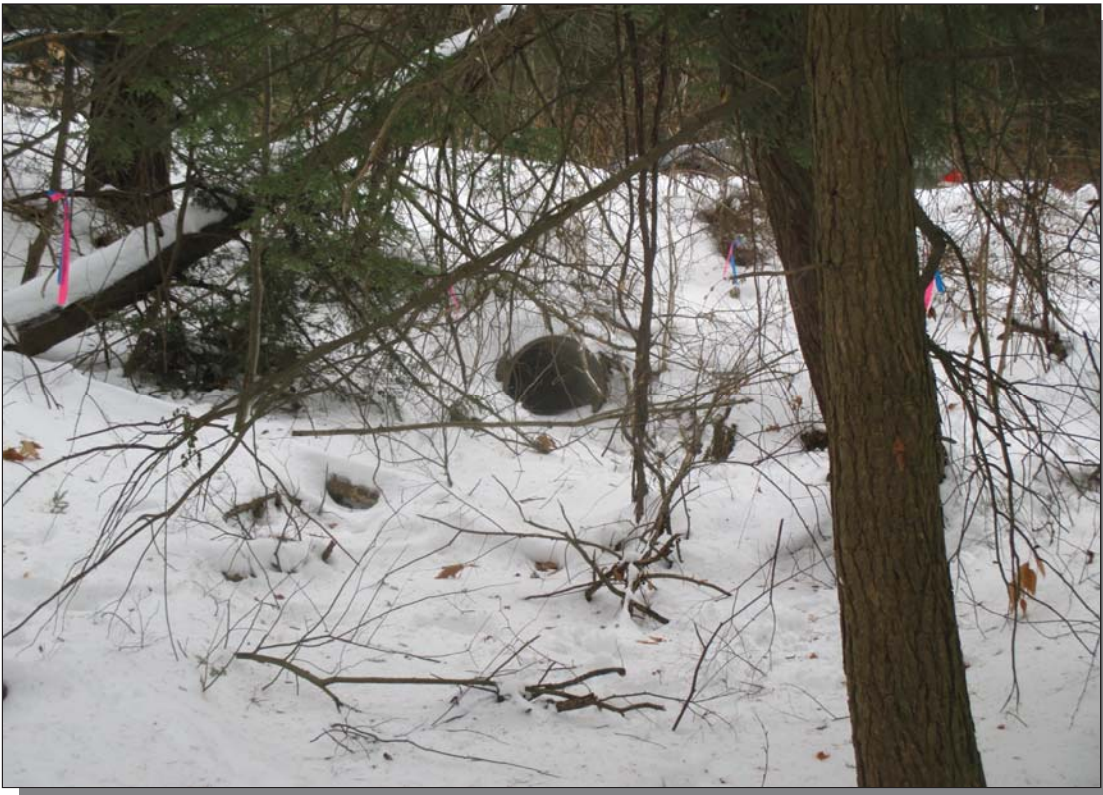
Photo 3: View of intermittent watercourse/30-inch RCP (JMM-1A-Series) (JMM photo taken 1/9/17); facing southwesterly
