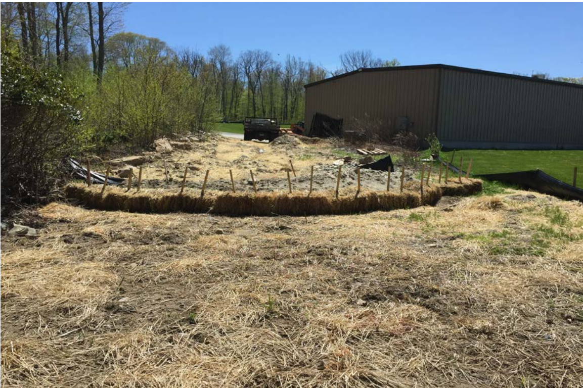
Photo 4: View of check dam leading to Wetland 6.
