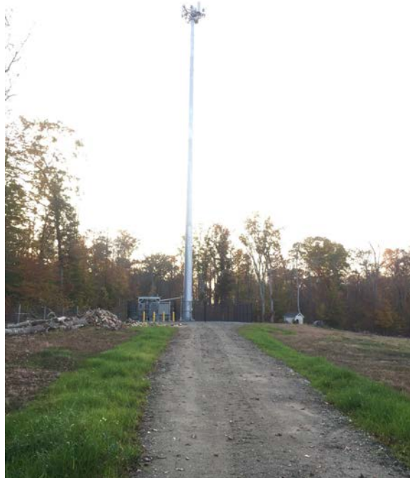
Photo 2: View of tower and compound area.
