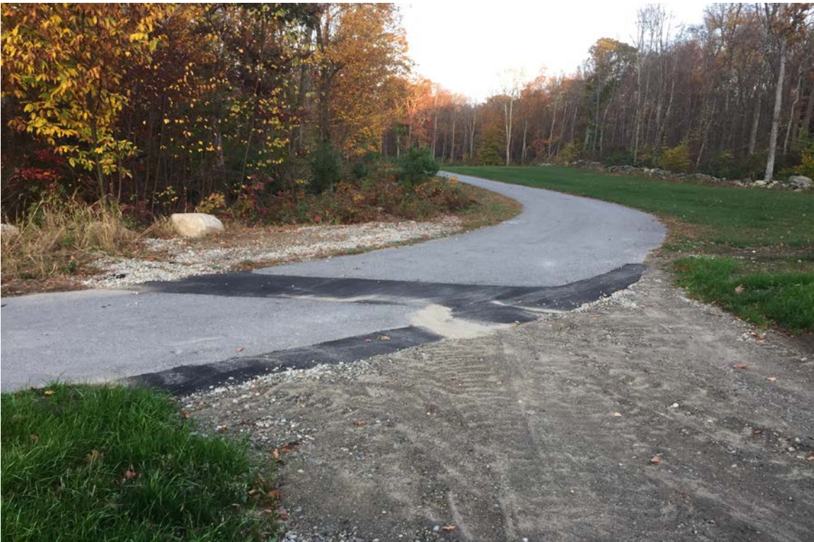
Photo 6: View of utility route crossing of existing paved access road.
