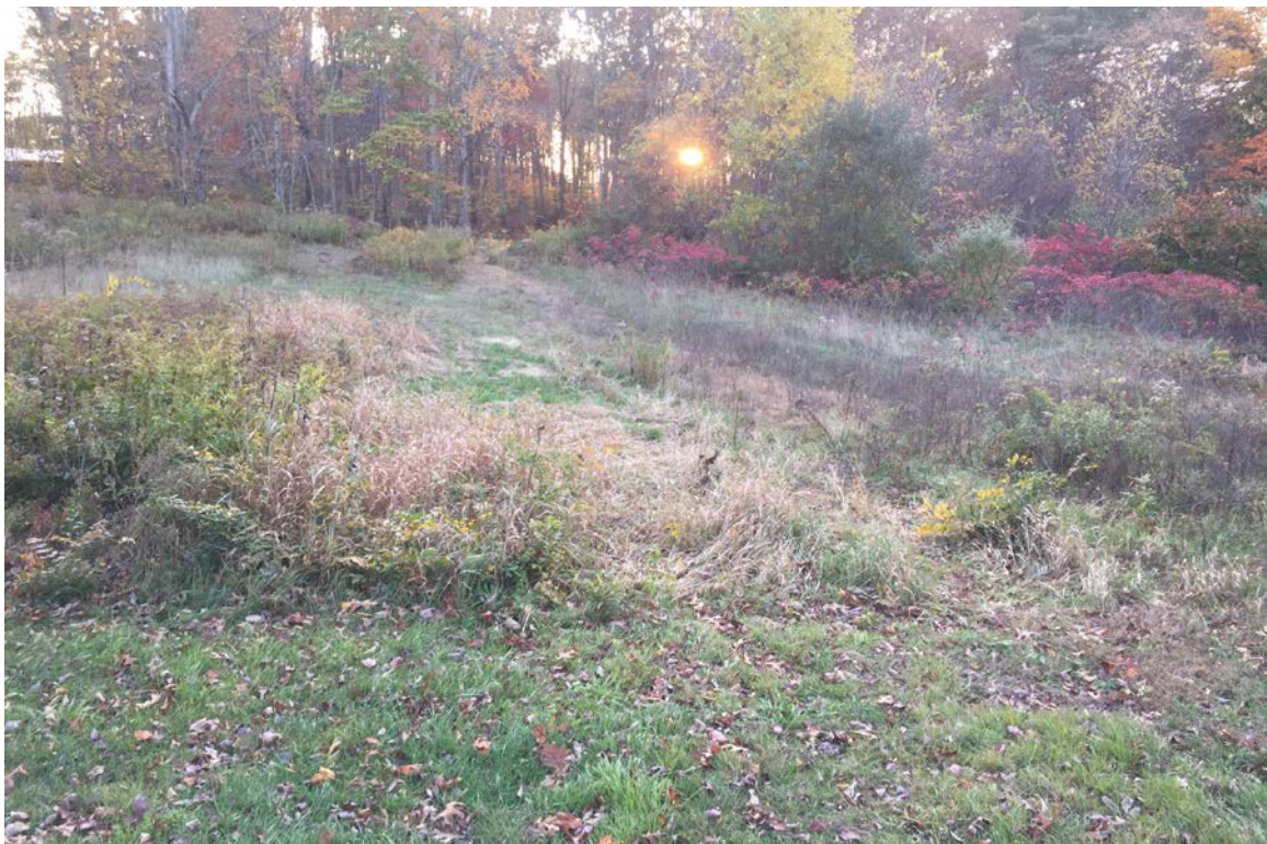
Photo 8: View of restored utility route/silt fence properly removed.
