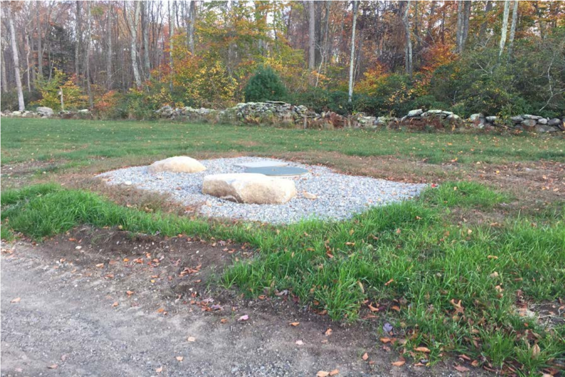
Photo 5: View of utility vault.
