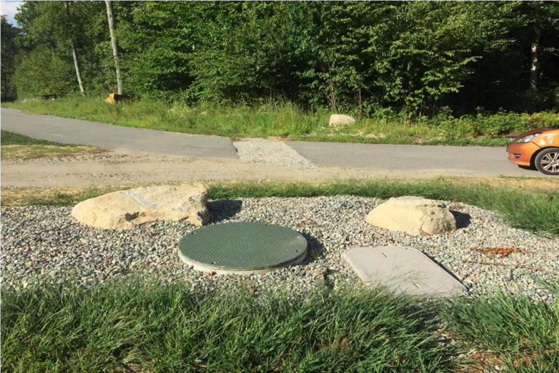
Photo 5: View of utility vault.
