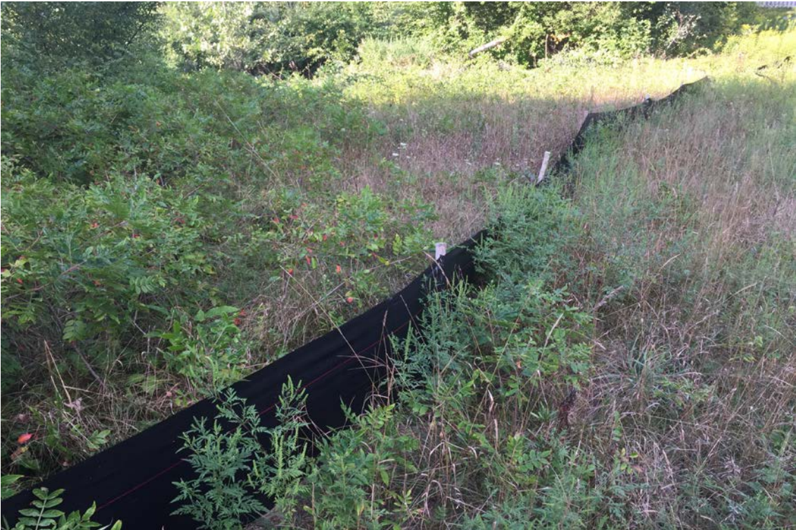
Photo 6: View of well-maintained silt fence.
