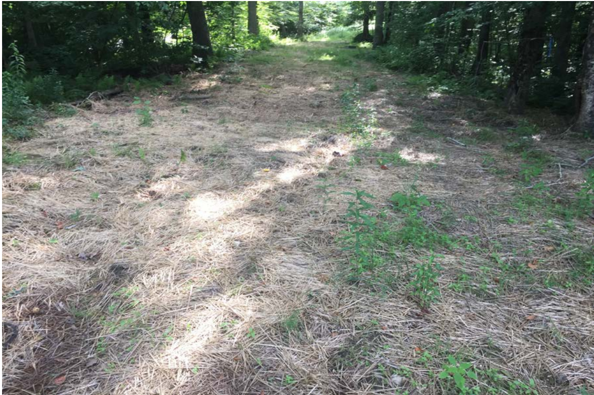
Photo 3: View of utility route wetland crossing partially stabilized.
