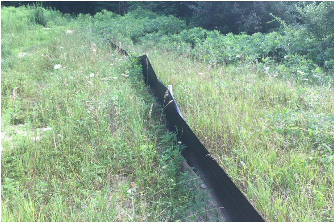
Photo 6: View of well-maintained silt fence.
