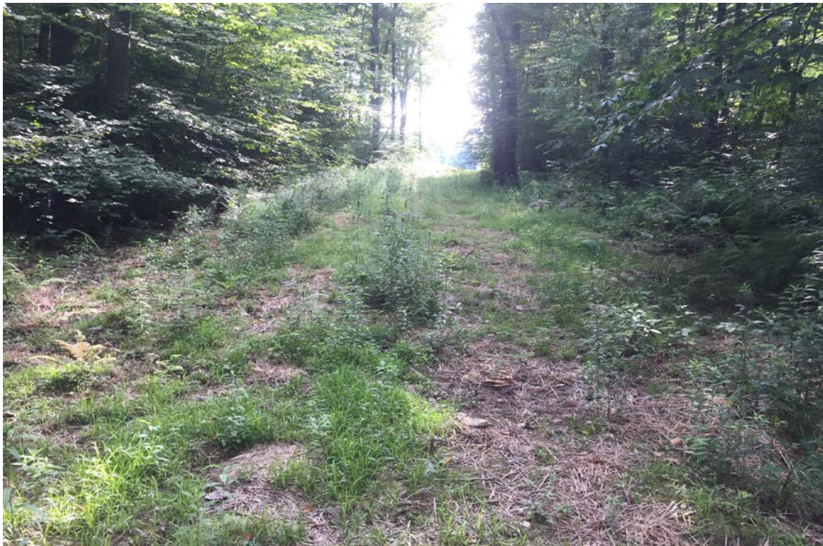
Photo 4: View of utility route wetland crossing stabilized with permanent vegetation.
