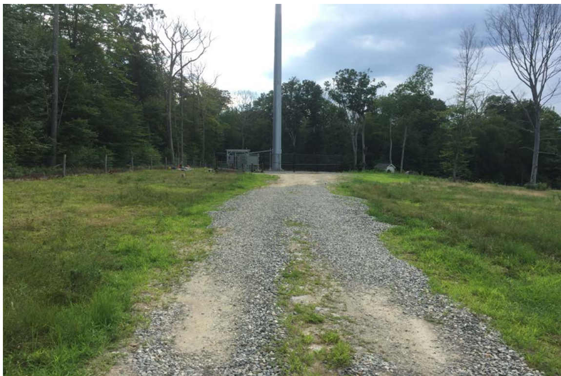
Photo 2: View of access road with compound area in background.
