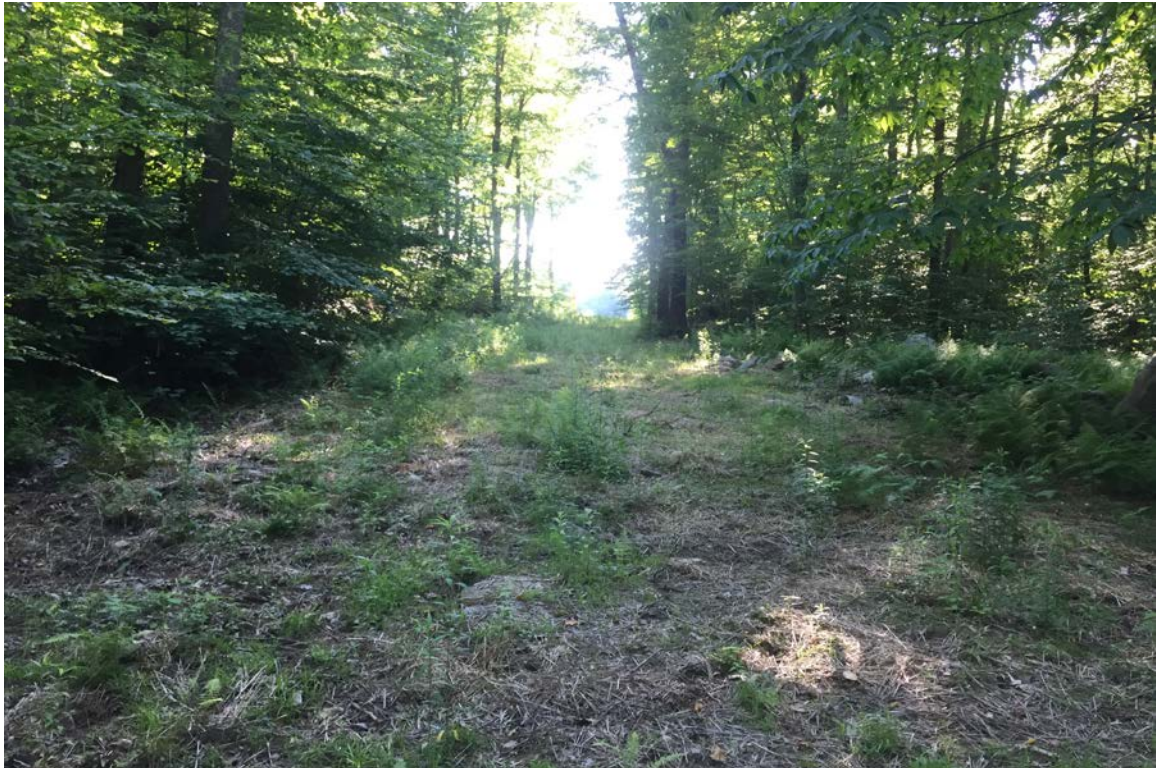
Photo 5: View of utility conduit wetland crossing post stabilization/seedling (note germination).
