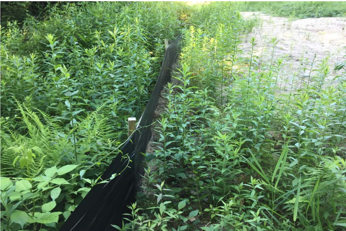
Photo 4: View of maintained silt fence.
