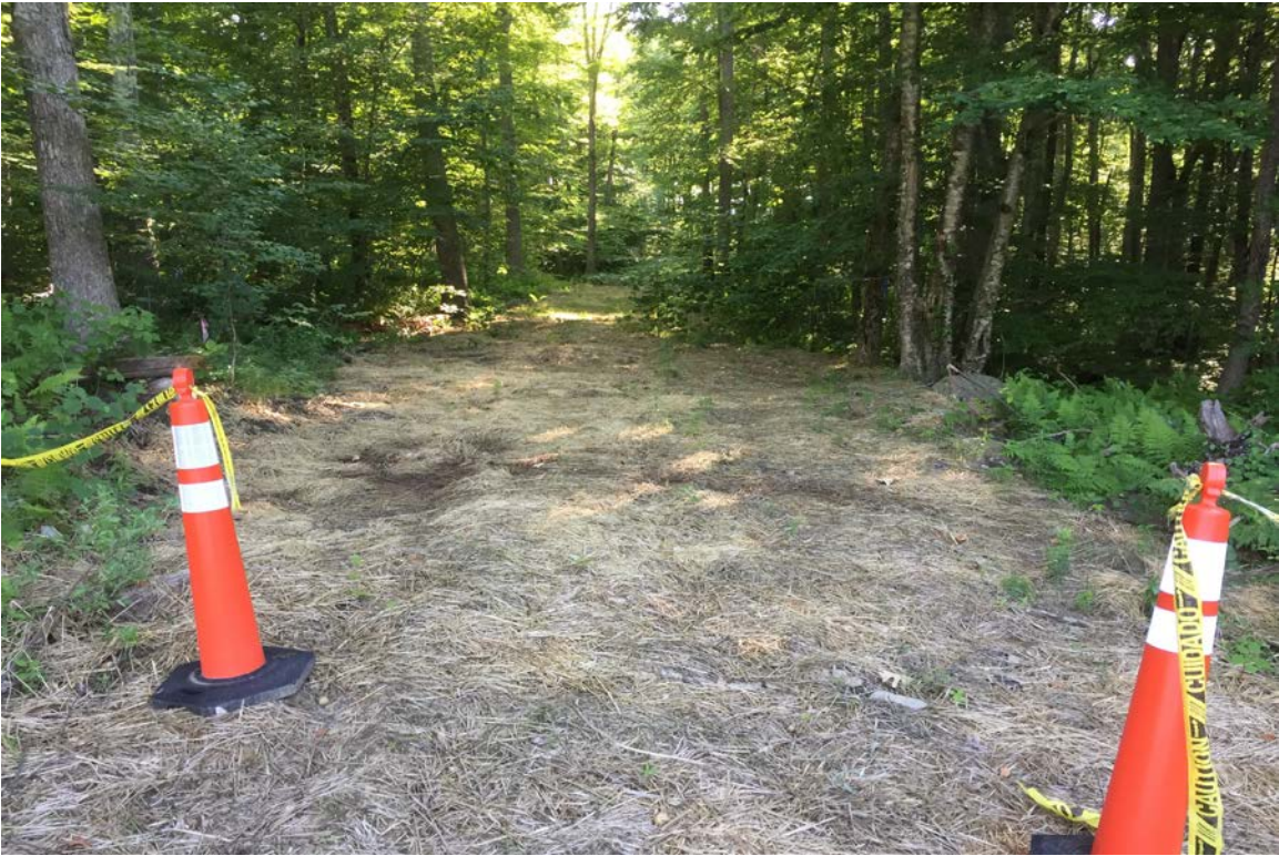
Photo 3: View of utility conduit wetland crossing.
