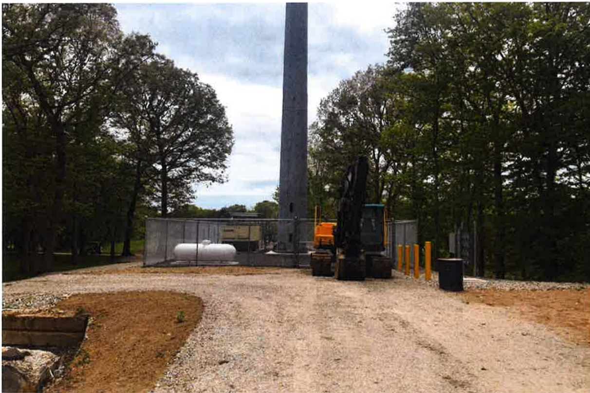
Photo 2: View of compound area/tower.
