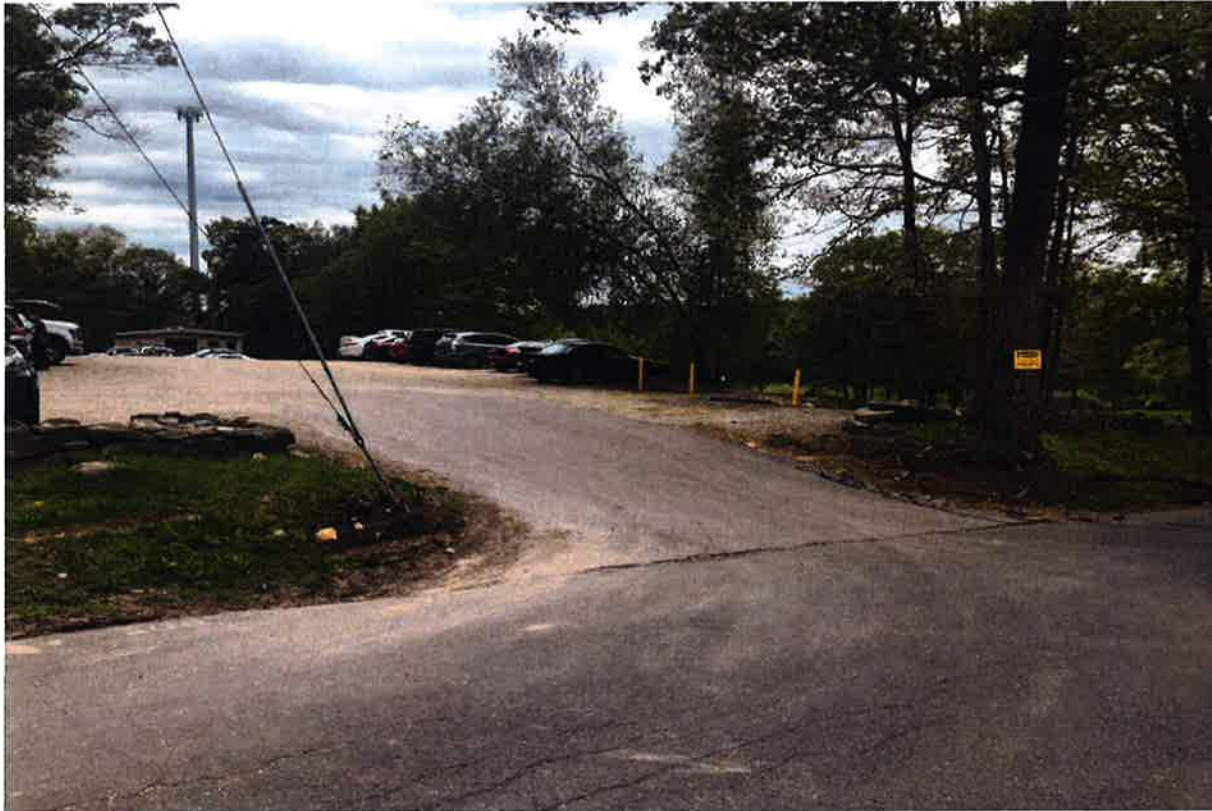
Photo 1: View of construction entrance off Folly Lane.
