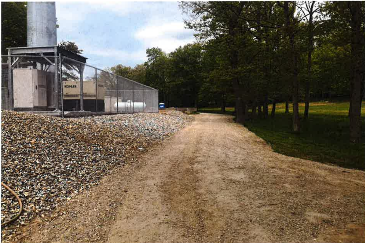
Photo 6: View of areas with silt fencing removed.
