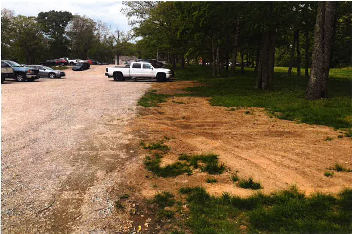
Photo 4: View of completed and backfilled electrical conduits.
