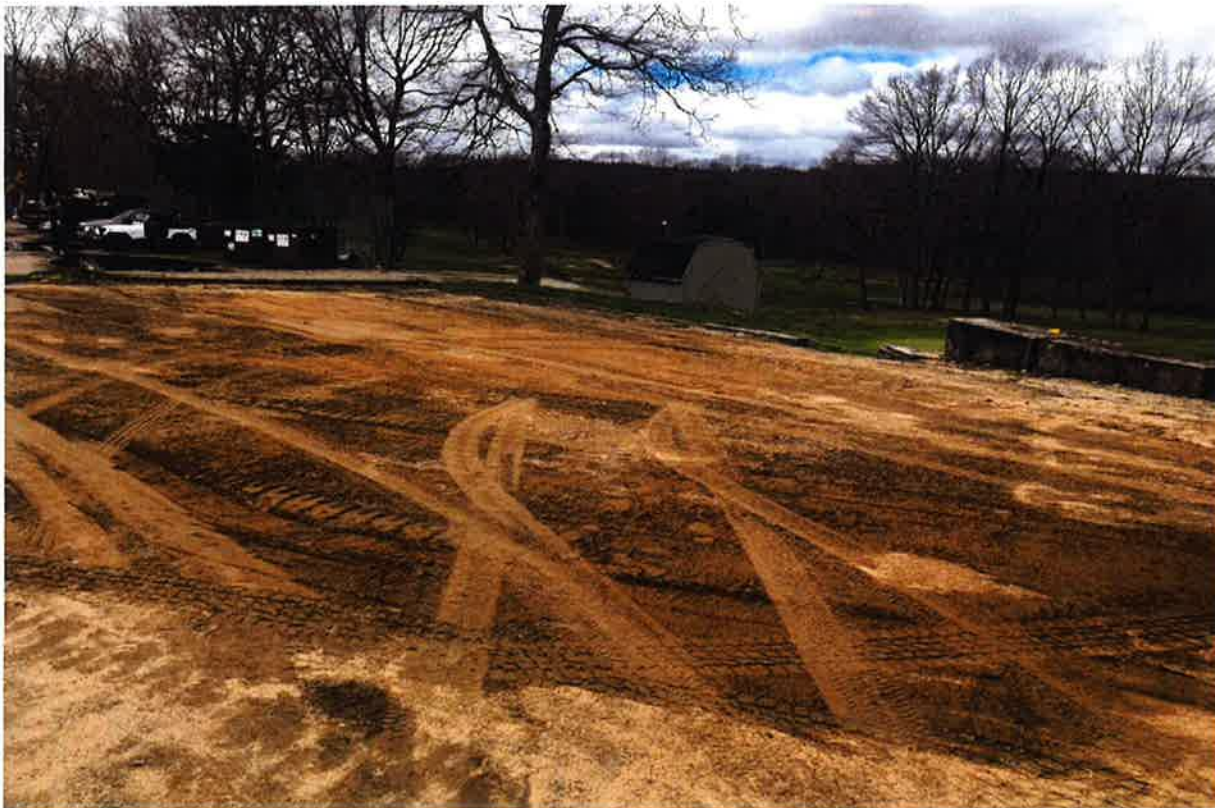
Photo 4: View of backfill stockpile removed.
