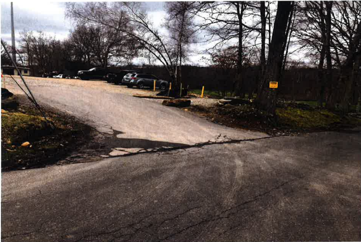
Photo 1: View of construction entrance off Folly Lane.
