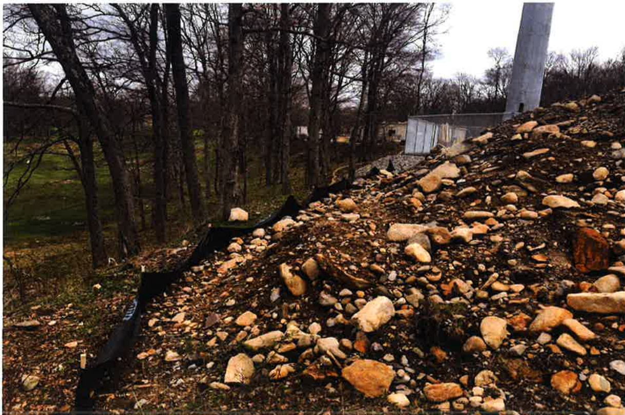
Photo 6: View of temporary excavation stockpile.
