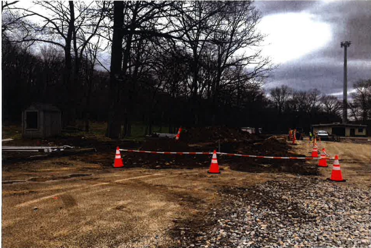
Photo 3: View of active trenching for electrical conduit construction.
