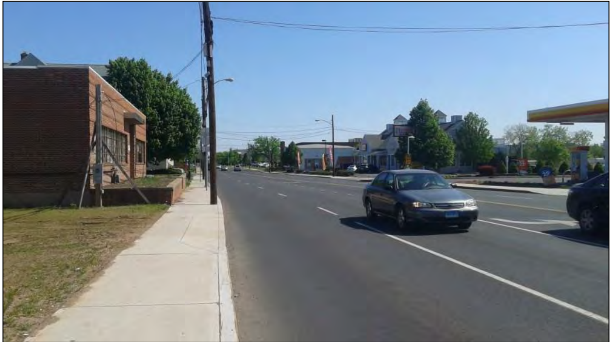
Photo 16. Overview photo of proposed project corridor facing north along New Park Avenue.
