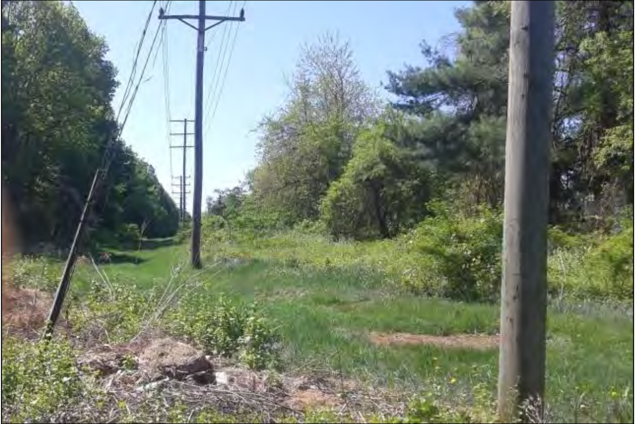
Photo 41. Overview photo of proposed project corridor facing south along an existing transmission line corridor.
