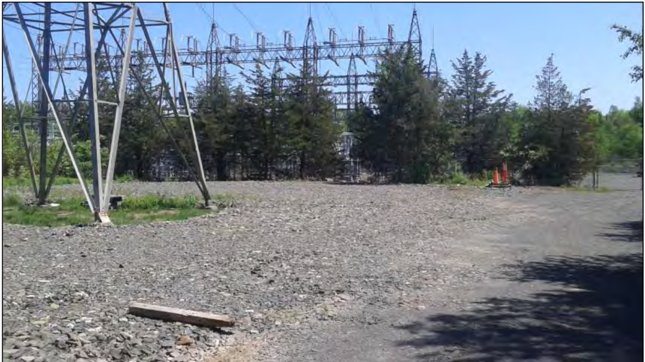
Photo 57. Overview photo of the Berlin Substation area facing east.
