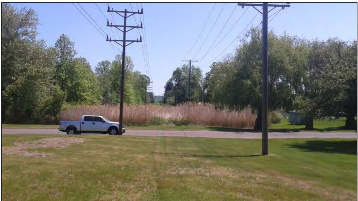
Photo 48. Overview photo of the Newington Substation facing east.
