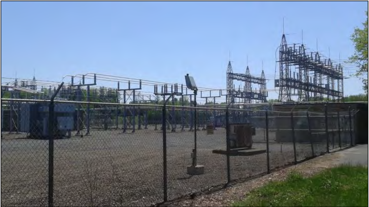
Photo 56. Overview photo of the Berlin Substation area facing southeast.
