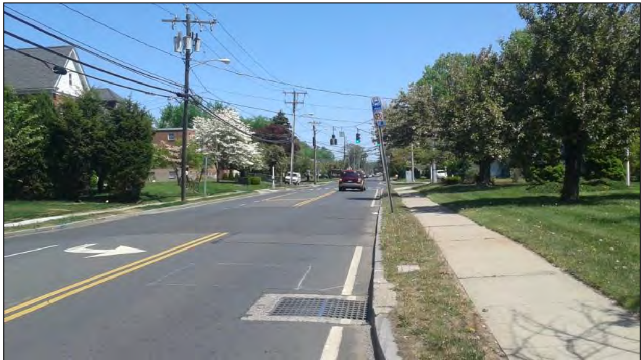
Photo 54. Overview photo of proposed project corridor facing north along Newington Road.
