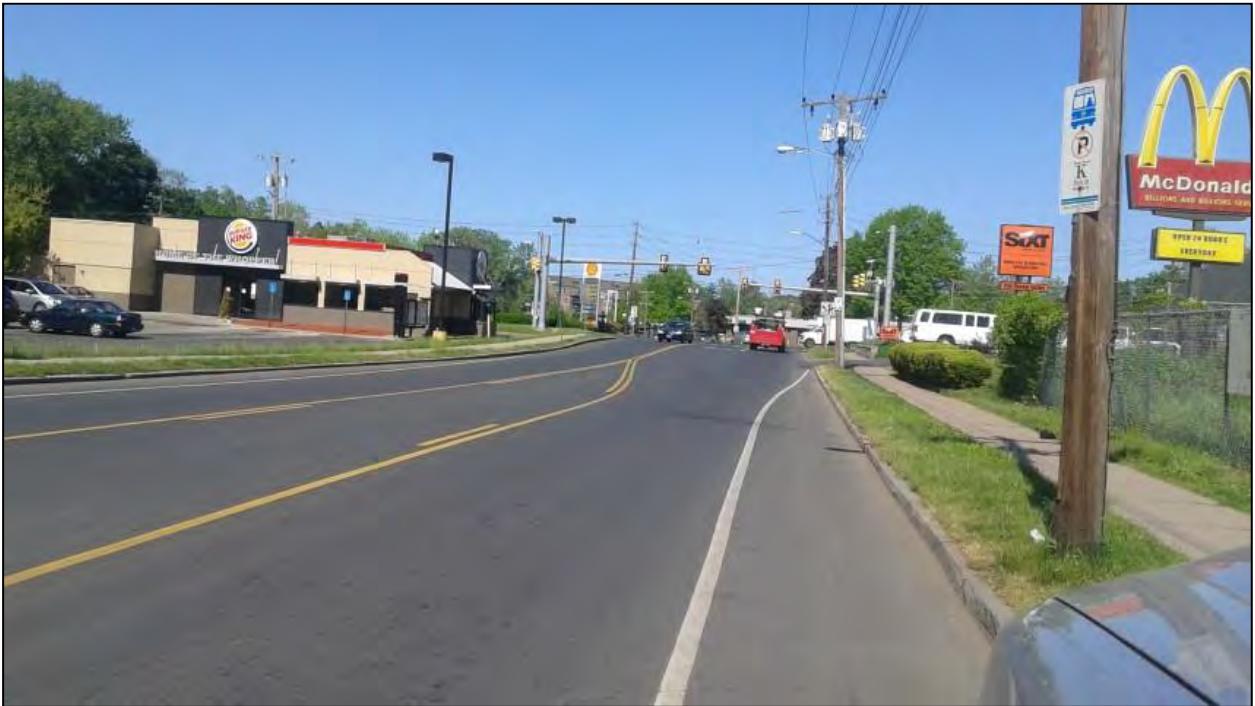
Photo 6. Overview photo of proposed project corridor facing west along Kane Street.
