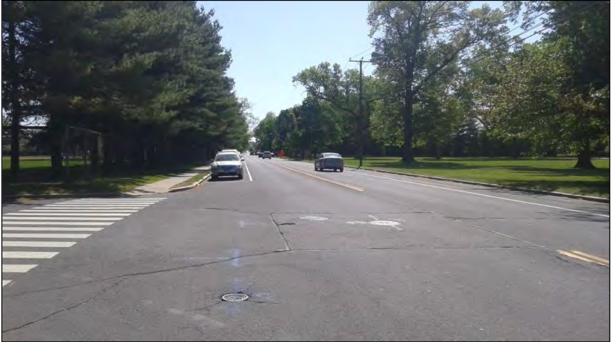
Photo 13. Overview photo of proposed project corridor facing east along Flatbush Avenue.
