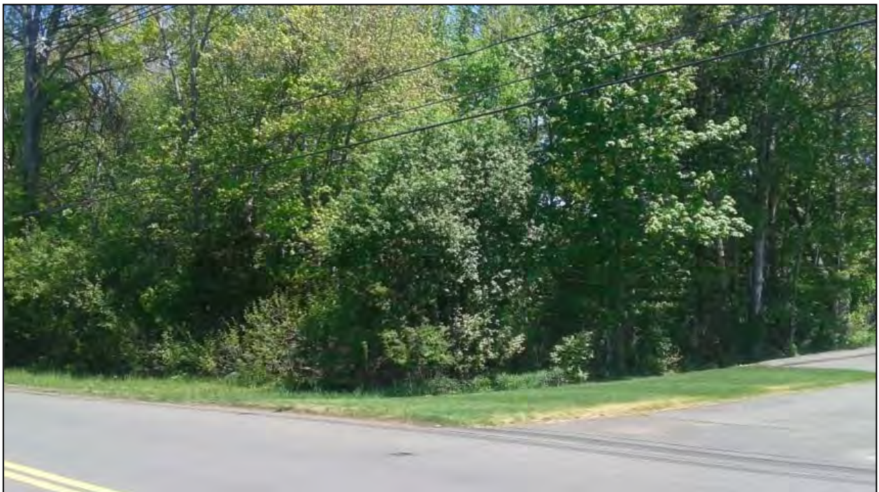
Photo 58. Overview photo of the Berlin Substation area facing northeast.
