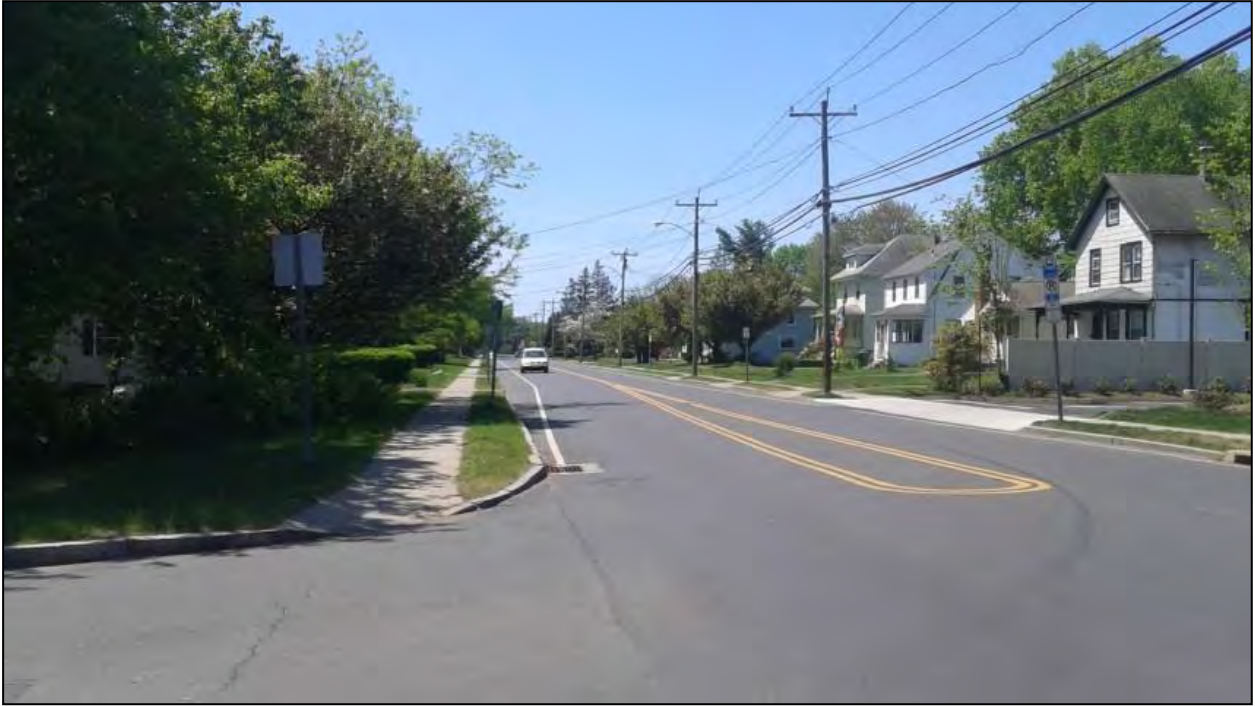
Photo 55. Overview photo of proposed project corridor facing north along Newington Road.
