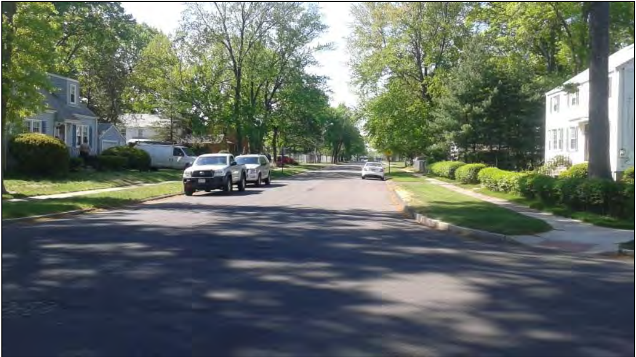
Photo 12. Overview photo of proposed project corridor facing south along Price Boulevard.
