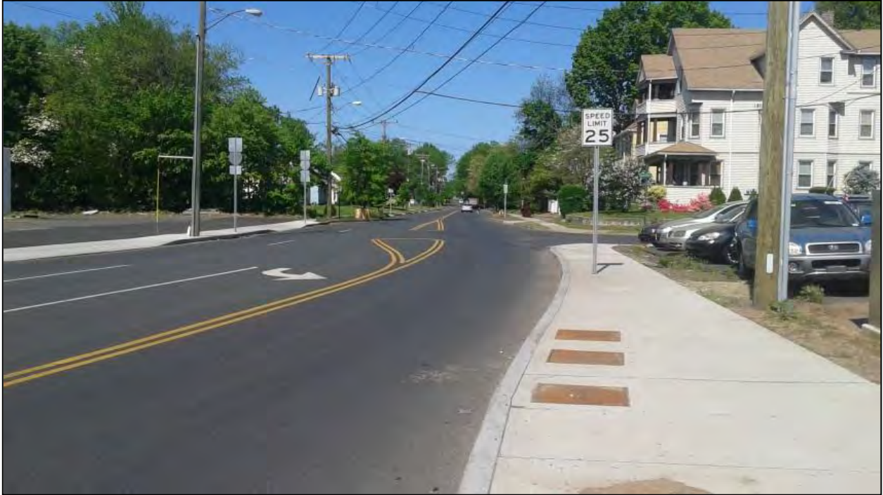
Photo 17. Overview photo of proposed project corridor facing west along Flatbush Avenue
