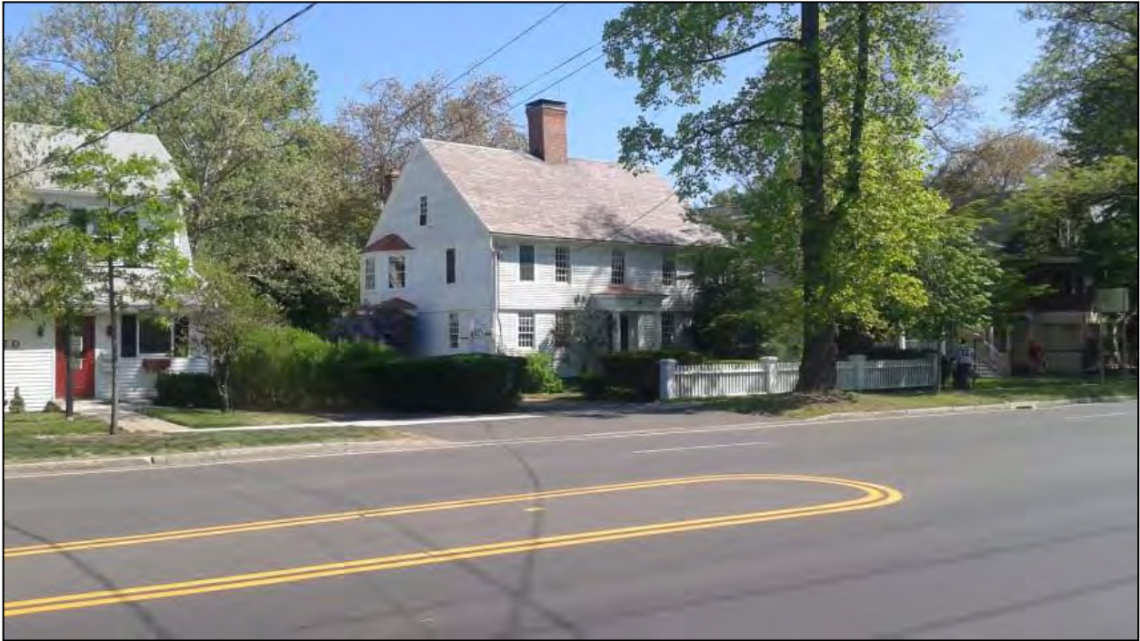
Photo 37. Overview photo of 1168 New Britain Avenue facing northeast (this house is listed on the National Register of Historic Places).
