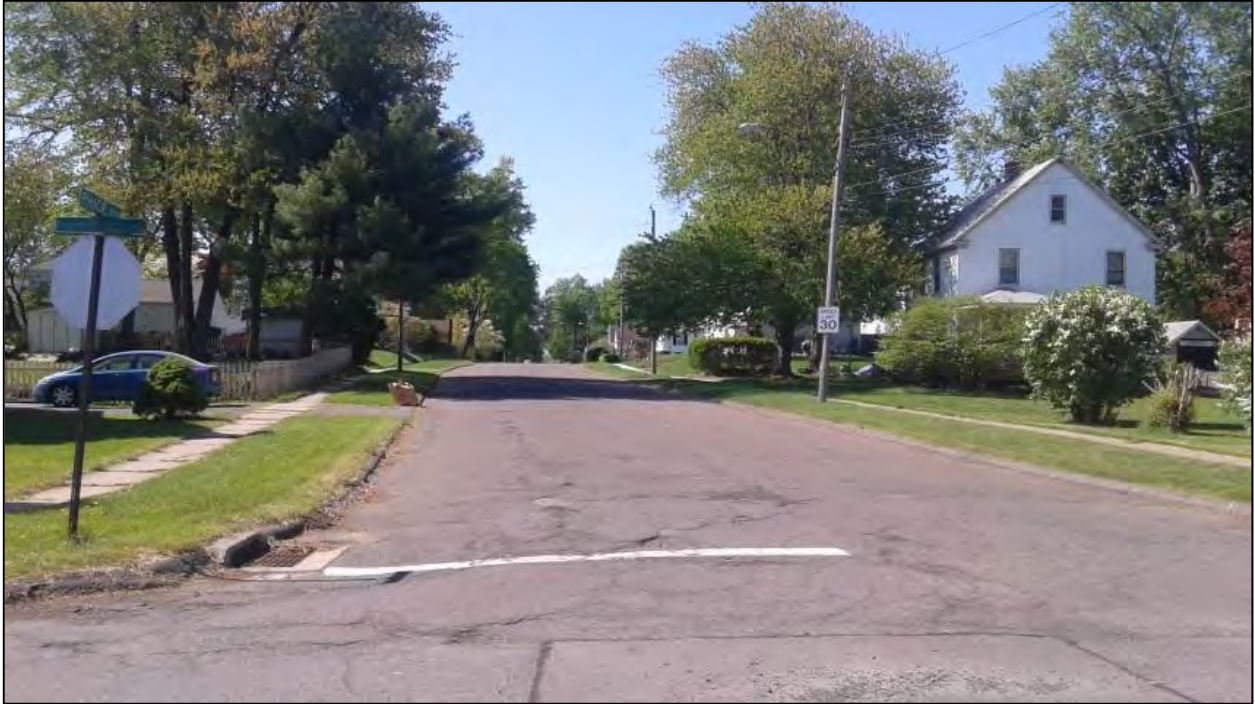
Photo 11. Overview photo of proposed project corridor facing south along Price Boulevard.
