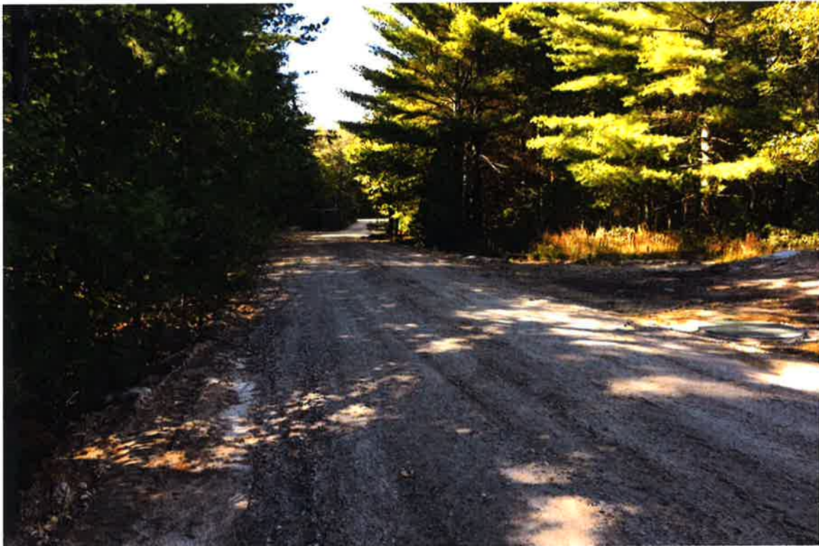
Photo 3: View of gravel access looking west.
