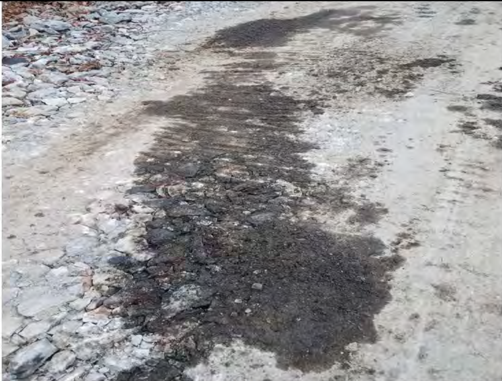
Photo 17: 12/22/2017, Watertown: Hydraulic oil release to the ground surface (access road) in the area of Str37.
