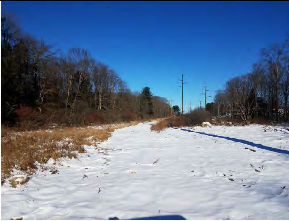
Photo 19: 12/28/2017, Litchfield: Map 28, W-E10, timber mat road and pads (Str78-Str80) removed, snow and ice covered wetland area.
