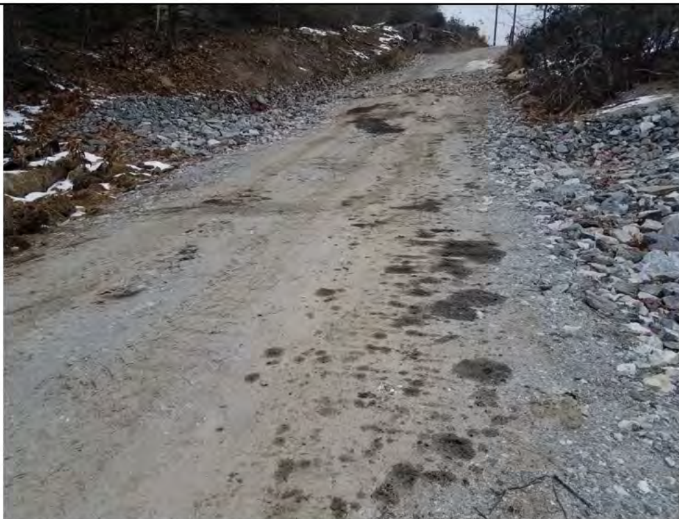
Photo 16: 12/22/2017, Watertown: Hydraulic oil release to the ground surface (access road) in the area of Str37.
