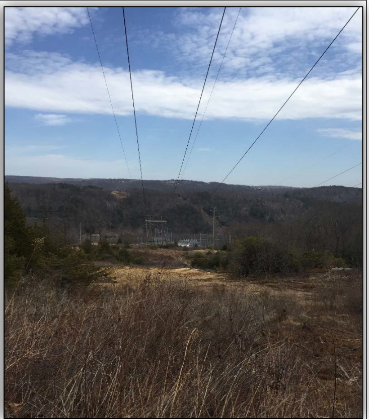
Photo 2: View of Frost Bridge Substation from Jericho Trail, Watertown. View to east along ROW from Trail crossing.
