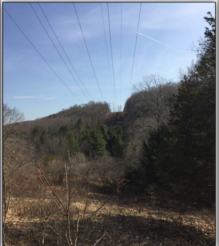
Photo 16: Northfield Brook Recreation Area, Thomaston. View to south (toward Walnut Hill Junction) from "Yellow" hiking trail crossing of Eversource ROW.
