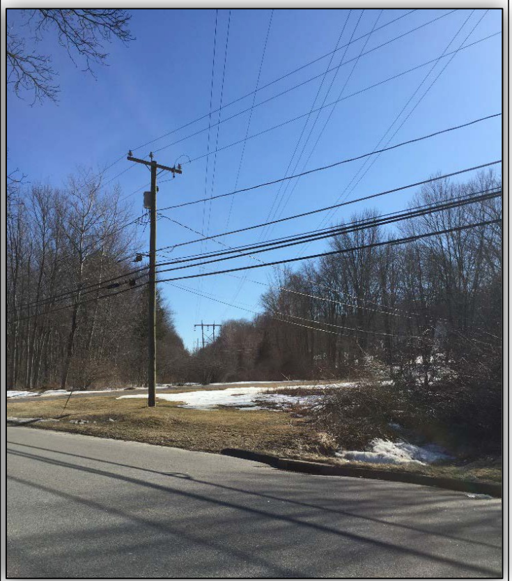
Photo 6: Walnut Hill Road, Thomaston. View to south from road crossing.
