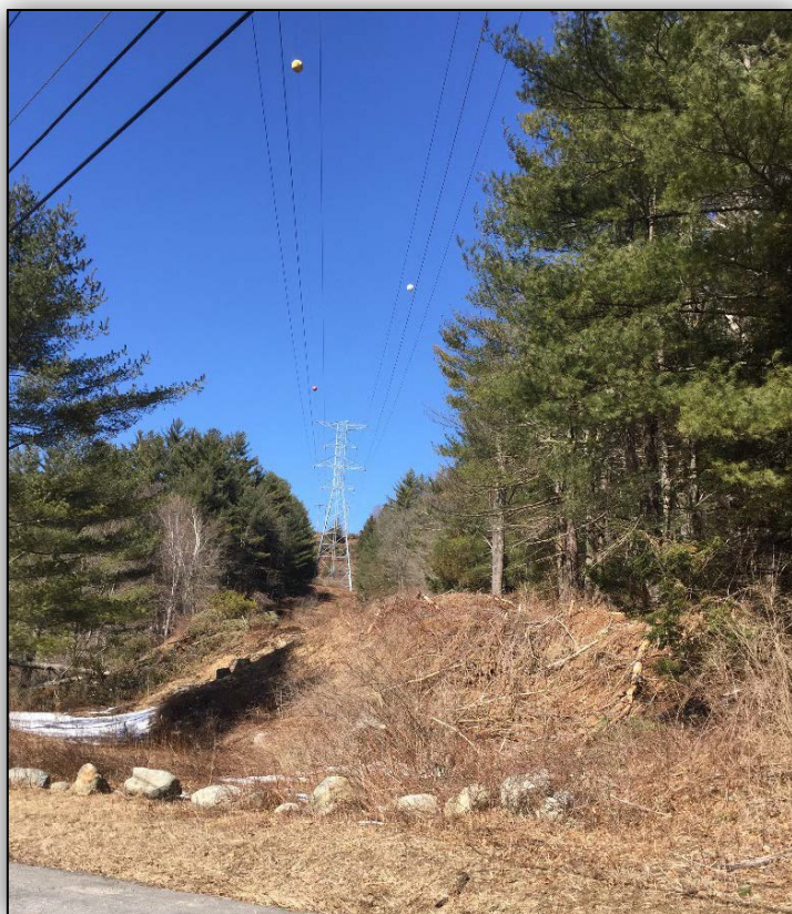
Photo 19: Valley Road, Harwinton. View to northeast of existing transmission line ROW.
