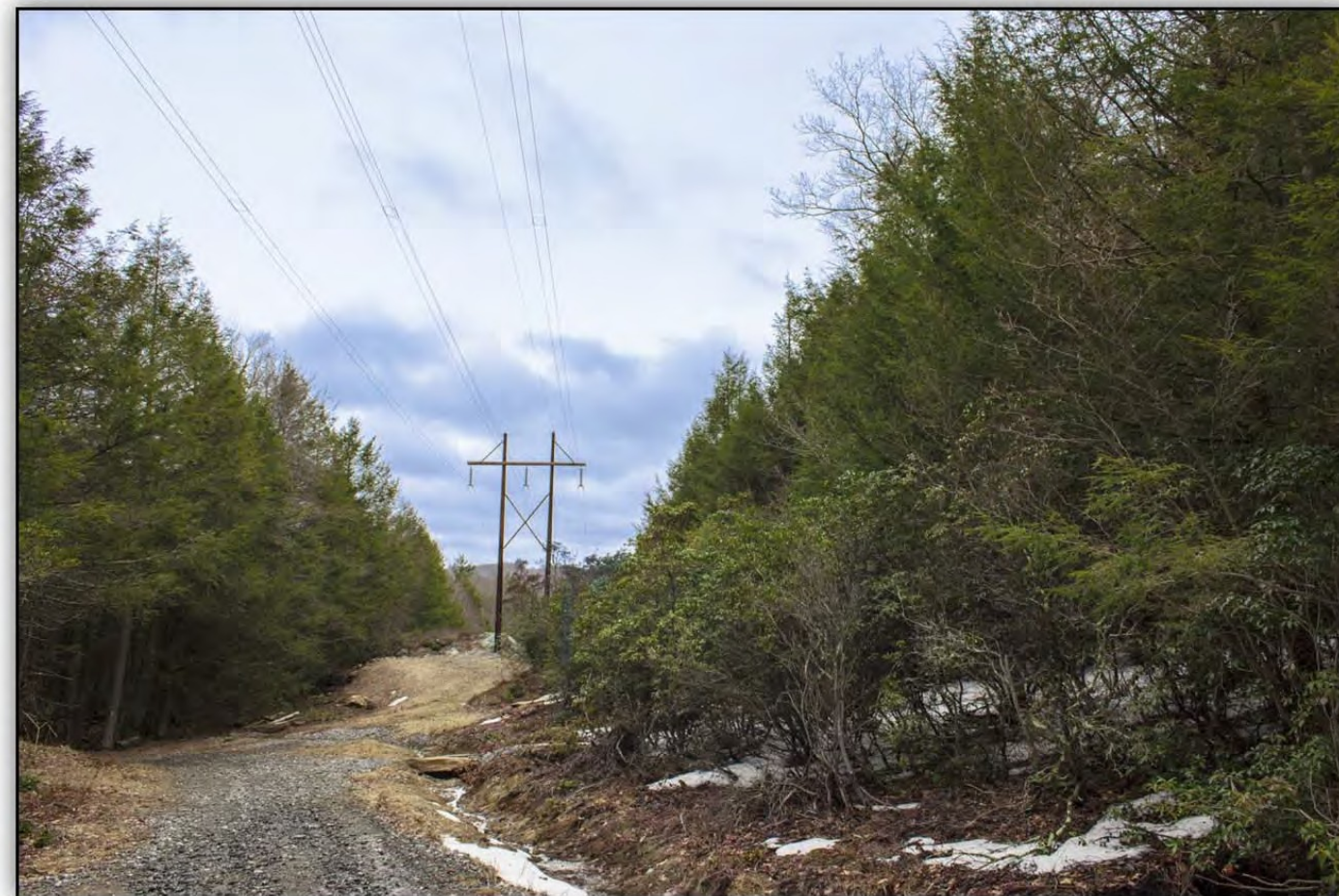
(Existing Transmission Right-of-Way – Leaf-off Condition)
