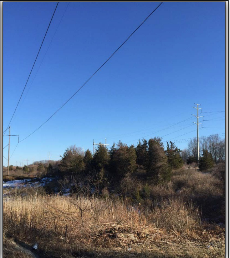
Photo 8: Nova Scotia Hill Road, Watertown. View southeast along ROW, toward Veterans Memorial Park, illustrating types of existing structures that occupy the ROW.
