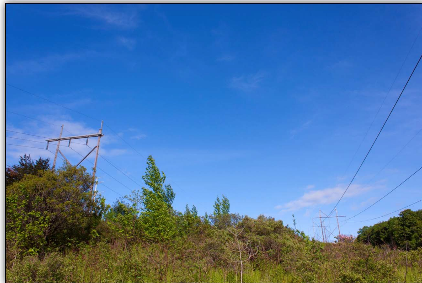
(Existing Transmission Right-of-Way – Leaf-on Condition)
