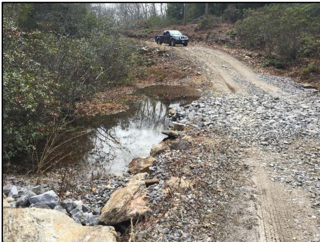
Photo 9: C20-1 is formed by the maintenance road embankment
