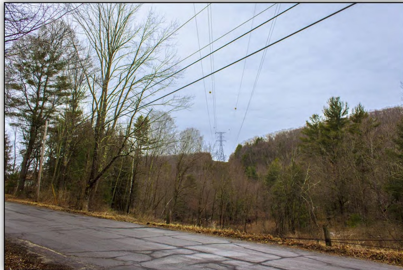
(Existing Transmission Right-of-Way – Leaf-off Condition)
