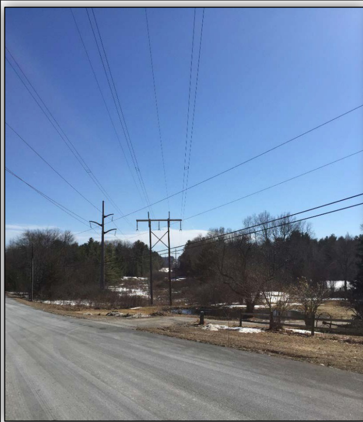
Photo 21: Wildcat Hill Road, Harwinton. View west along ROW near Campville Substation.
