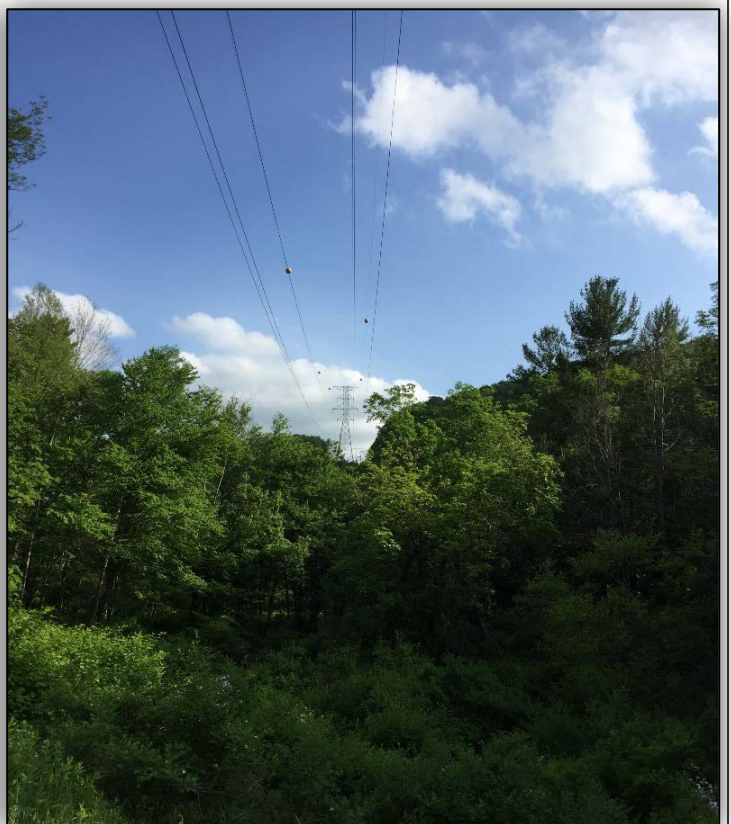
Photo 16: Valley Road, Harwinton. View to southwest of existing transmission line ROW, looking across Naugatuck River toward State Route 8.
