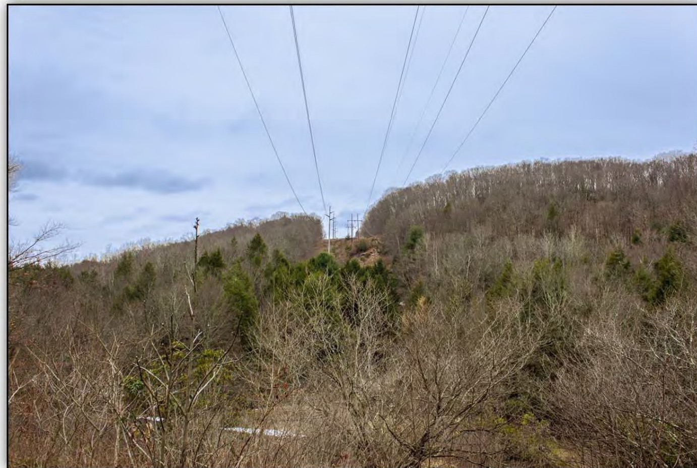
(Existing Transmission Right-of-Way – Leaf-off Condition)
