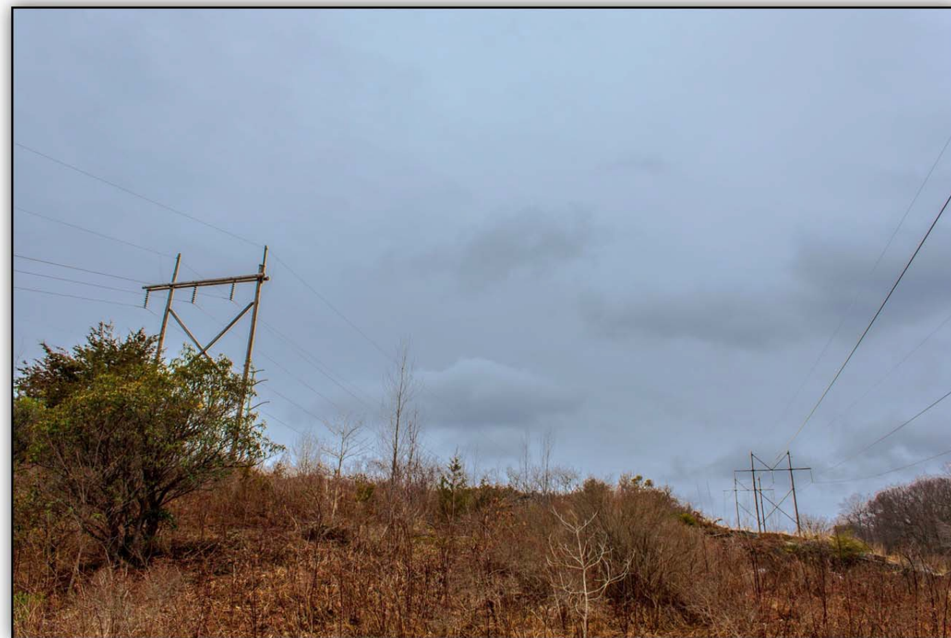
(Existing Transmission Right-of-Way – Leaf-off Condition)
