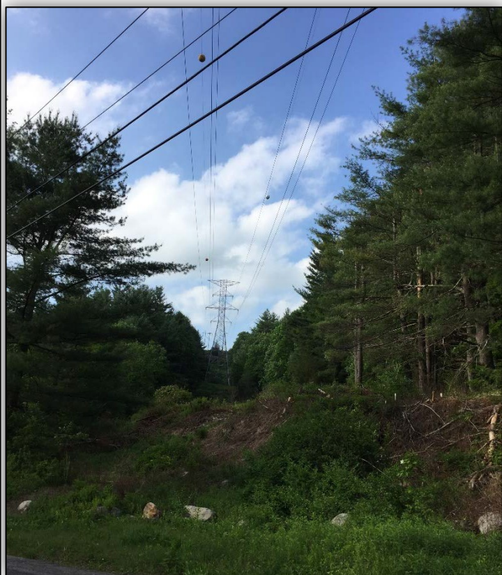
Photo 15: Valley Road, Harwinton. View to northeast of existing transmission line ROW and double-circuit steel lattice tower to be replaced.
