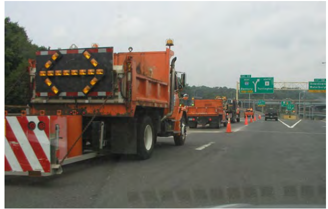
Construction on Route 8N before I-84 interchange
