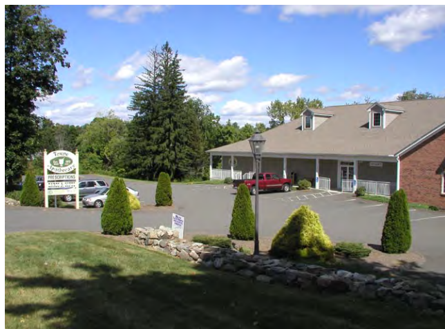
Commercial Building, Bethlehem
