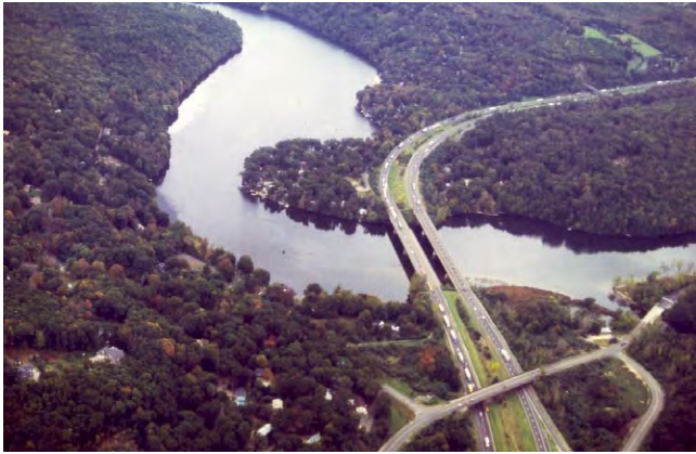
I-84 Crossing the Housatonic River, Southbury
