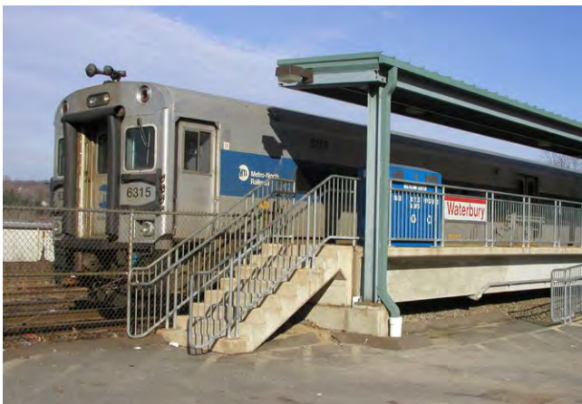
Train Station, Waterbury
