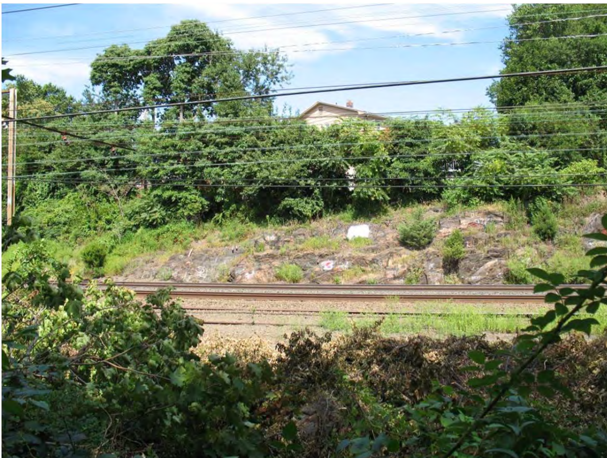
2. View north at active rail line that abuts the norther Site boundary.
