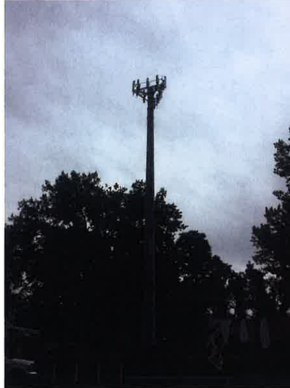
Photo 3: View of tower looking east.
