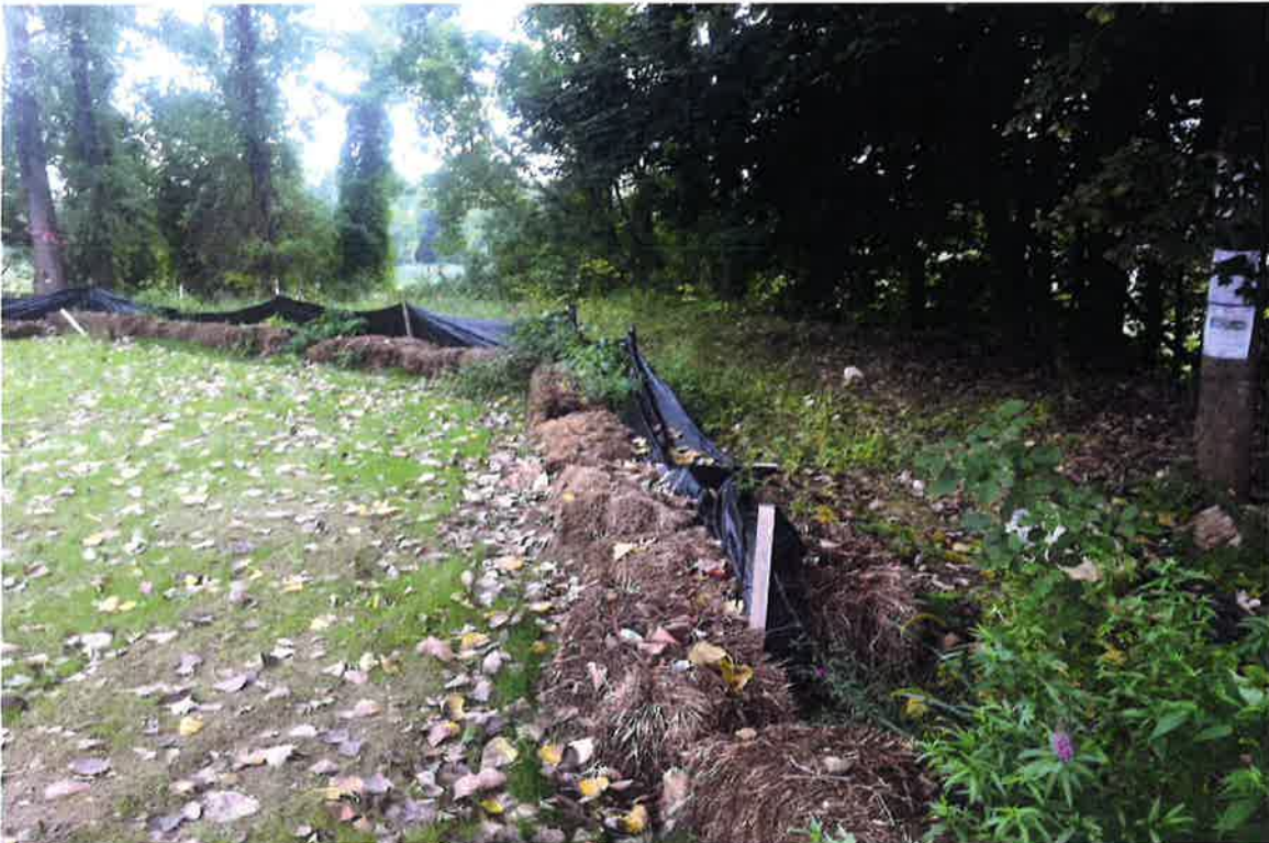
Photo 2: View of silt fence/ hay bale perimeter looking south.
