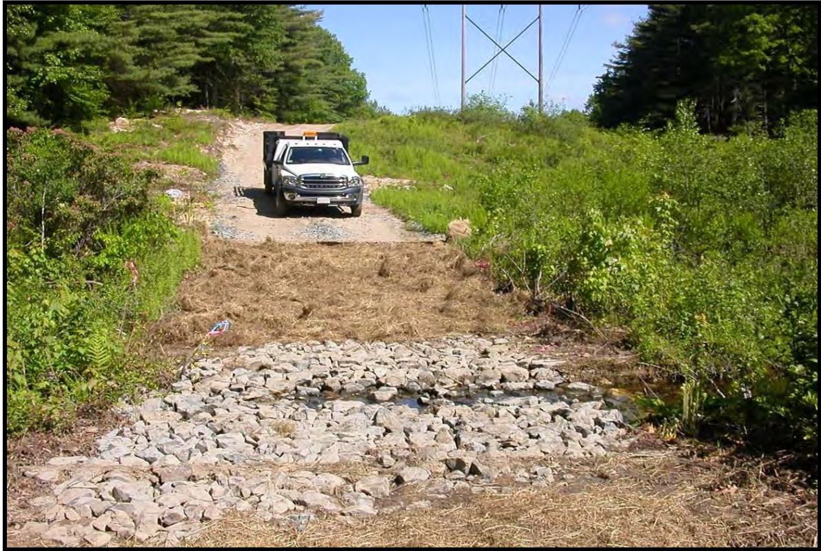
Intermittent stream crossing with angular stone.
