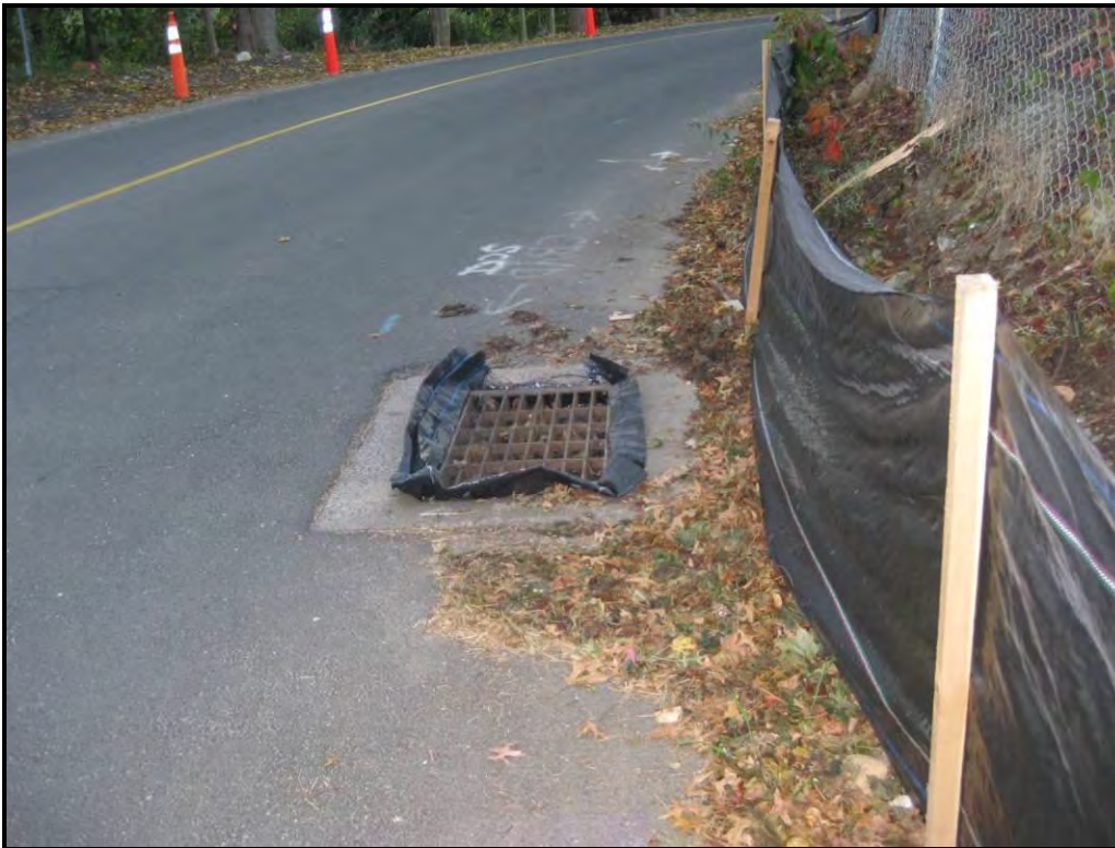
Catchbasin protected from sedimentation by filter fabric.
