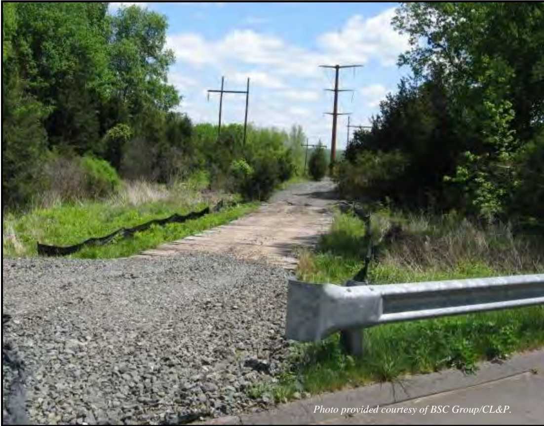
Construction entrance track pad.
