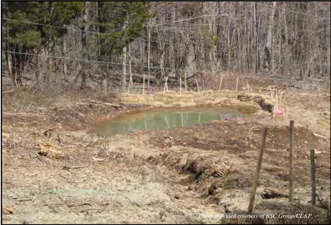
Sedimentation basin with hay bale filters.
