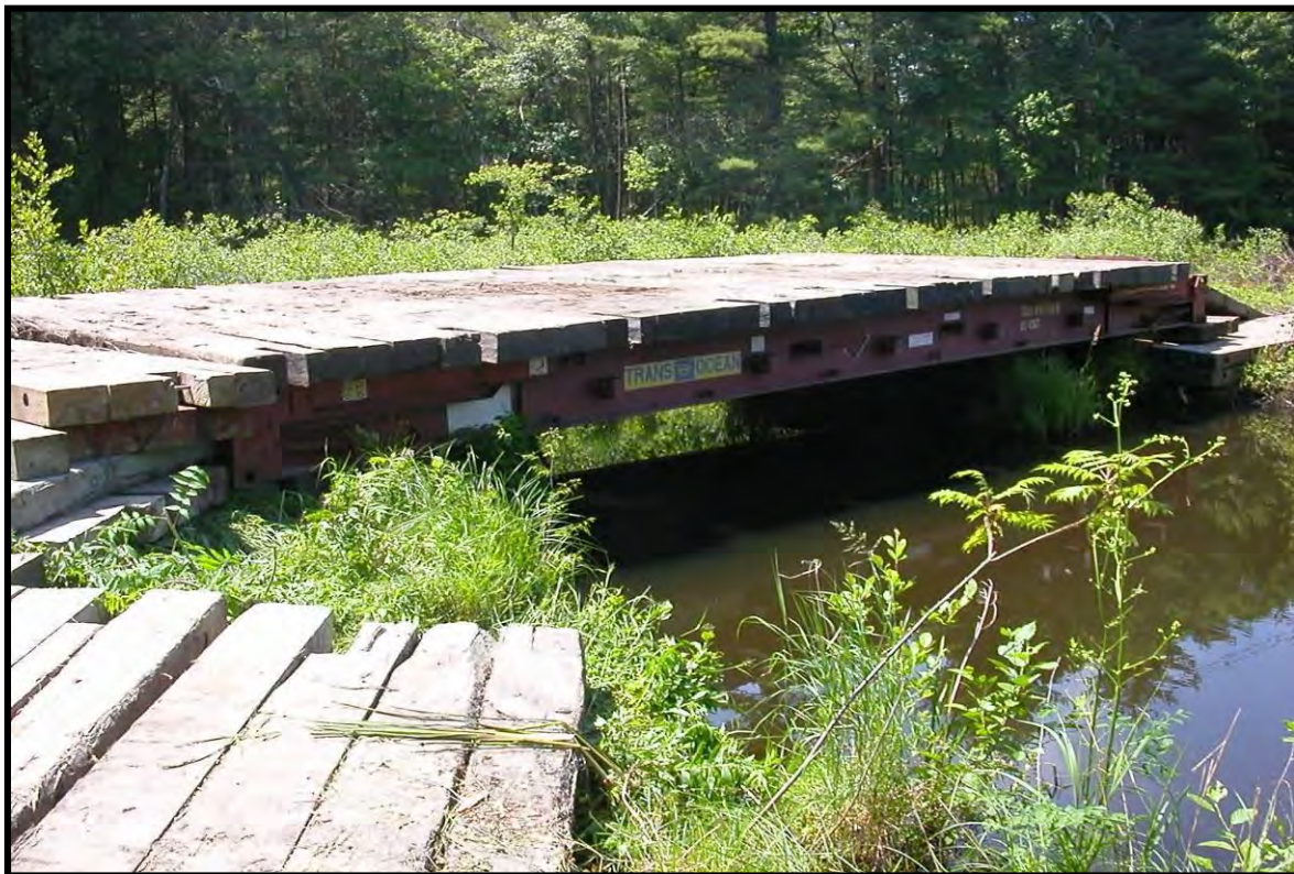
Rail car frame bridge crossing.
