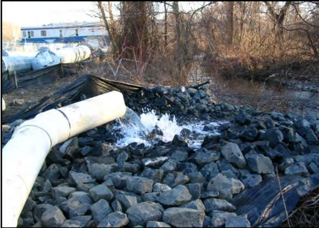
Riprap underlain by geotextile fabric
