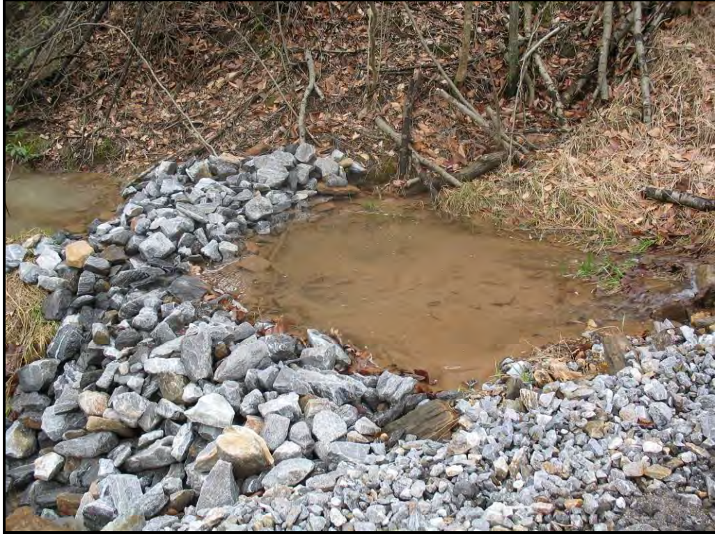
Stone check dam at construction site.
