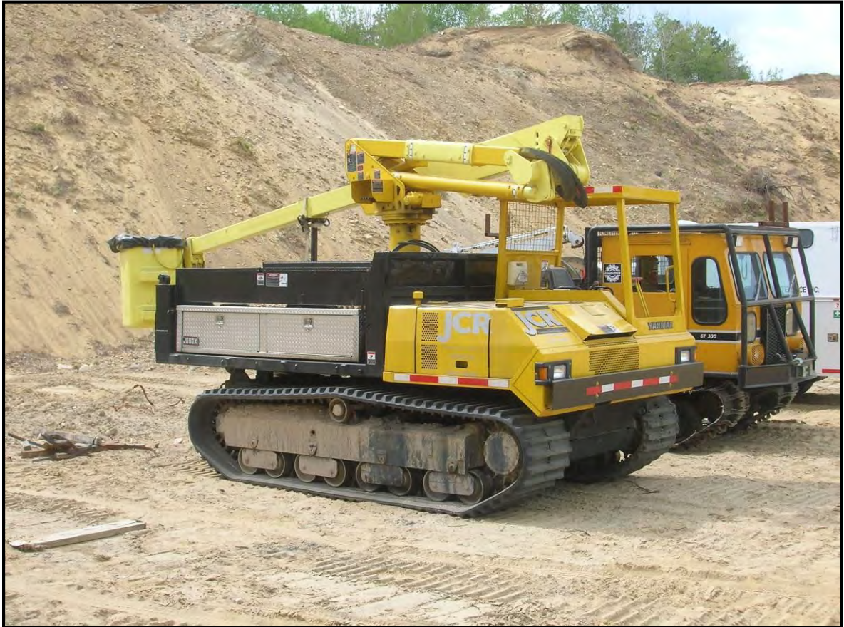
Equipment with rubberized tracks.
