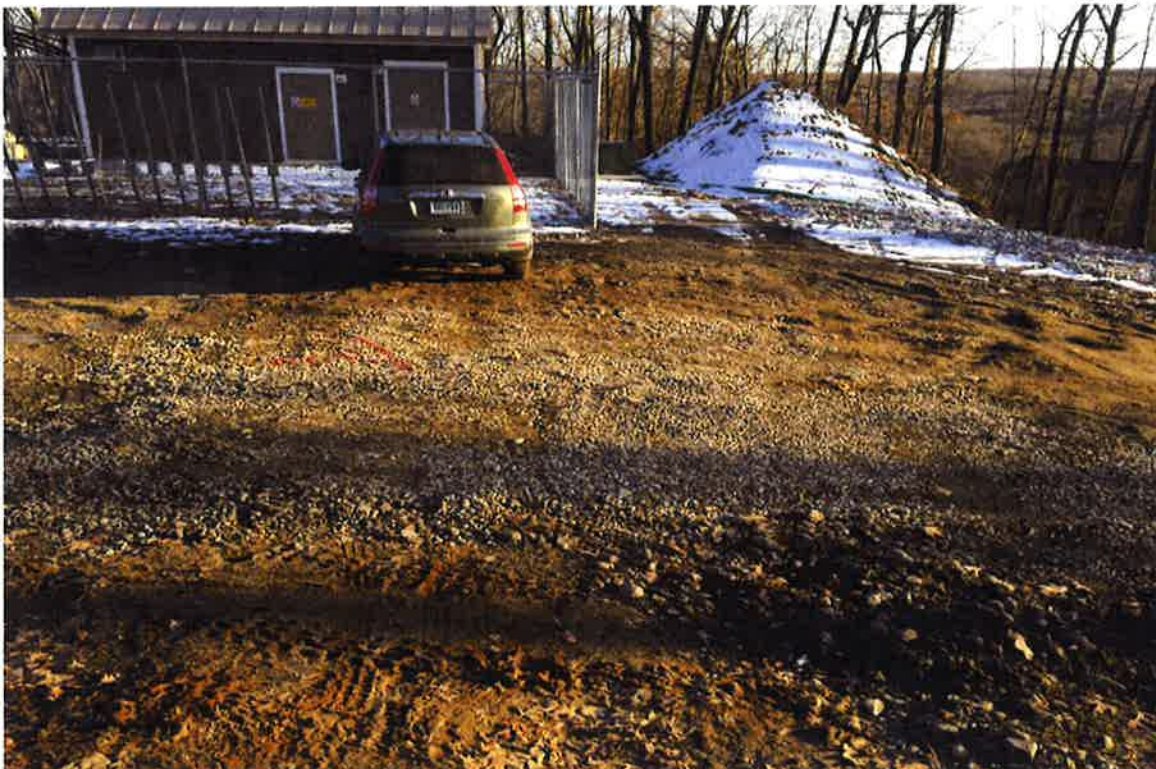
Photo 4: View of top of access drive top dressed with gravel looking south.
