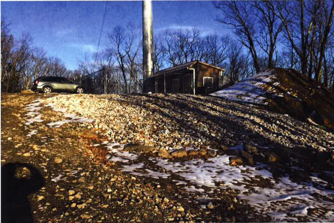
Photo 1: View of rock armored slope looking east.
