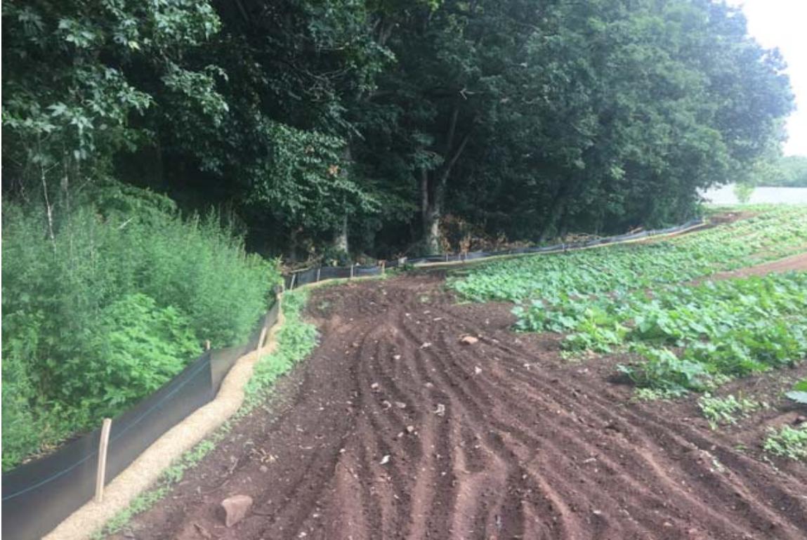
Photo 1: View of silt fence barrier looking east.
