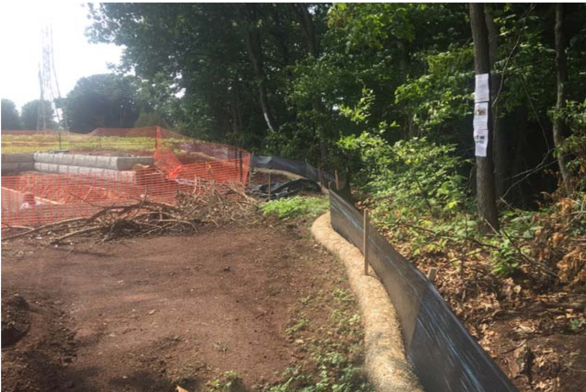
Photo 2: View of silt fence barrier looking west at north side of compound.
