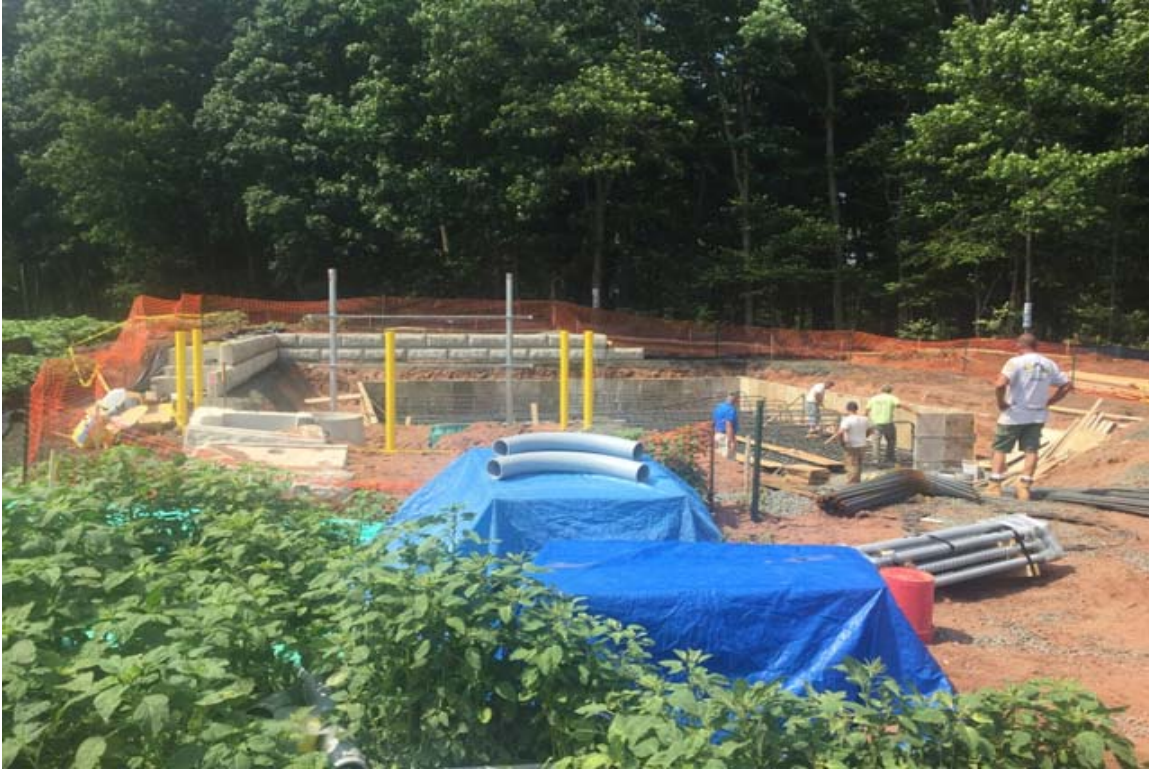
Photo 5: View of compound area looking north; tower foundation rebar being installed.
