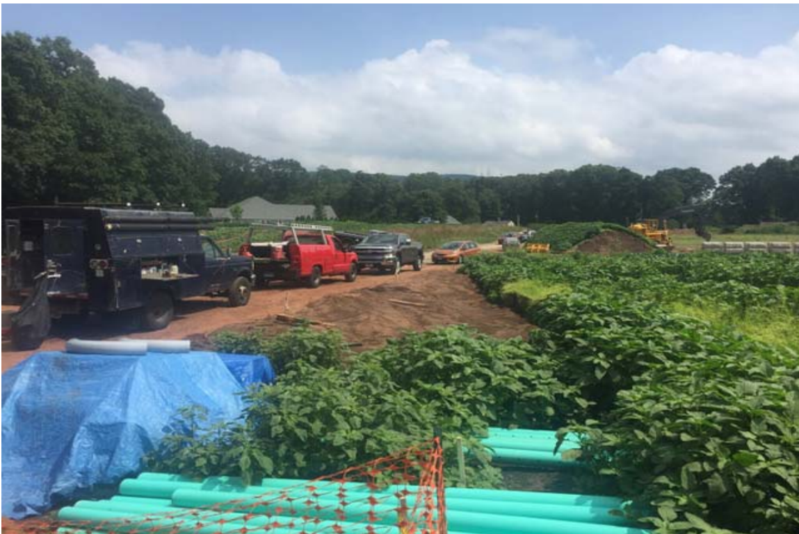
Photo 4: View of access road looking south from southwest corner of compound.
