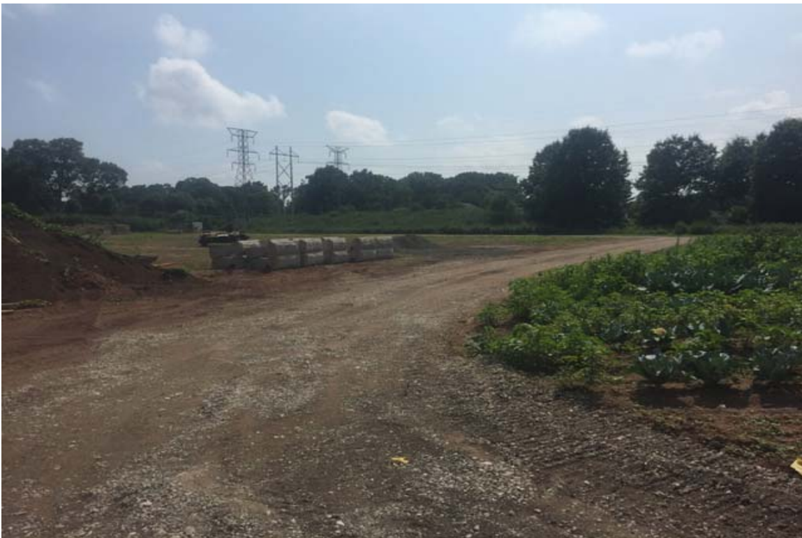
Photo 6: View of existing access road looking west.
