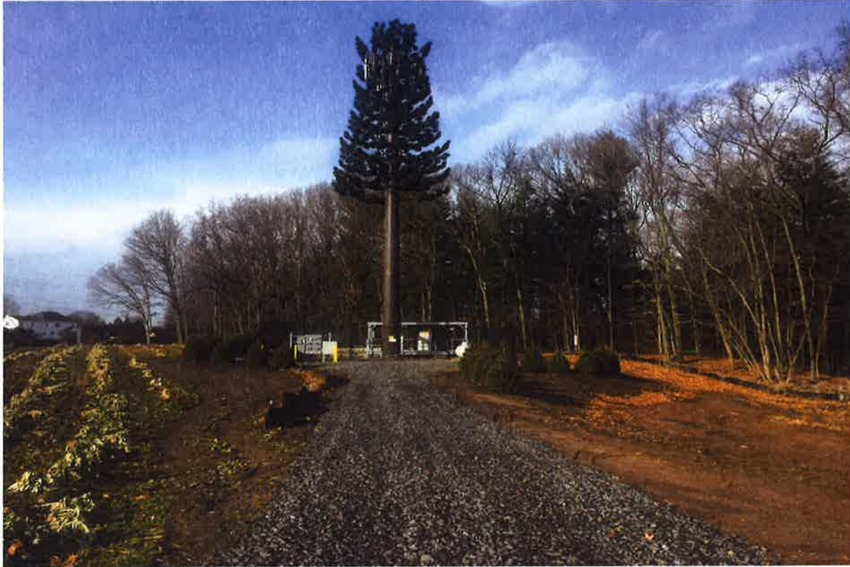
Photo 7: View of tower and compound area looking north.
