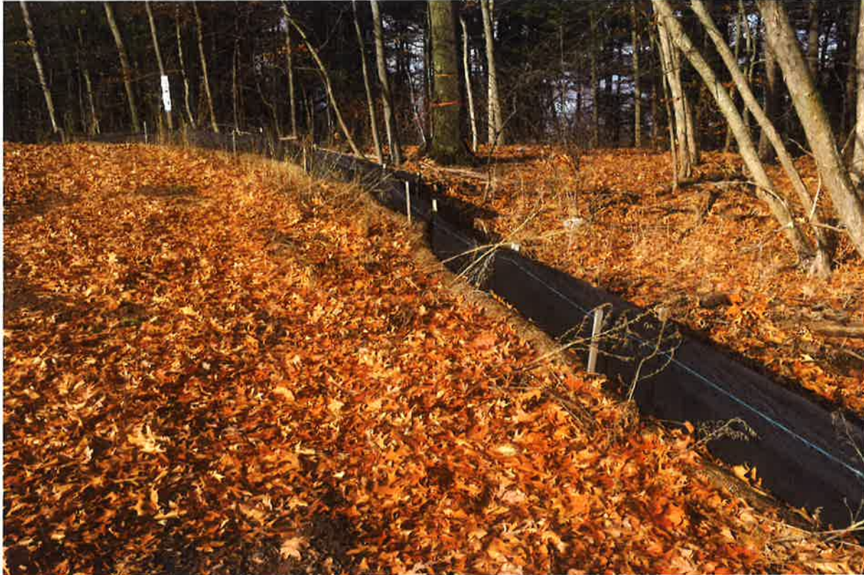
Photo 5: View of silt fence looking northwest.
