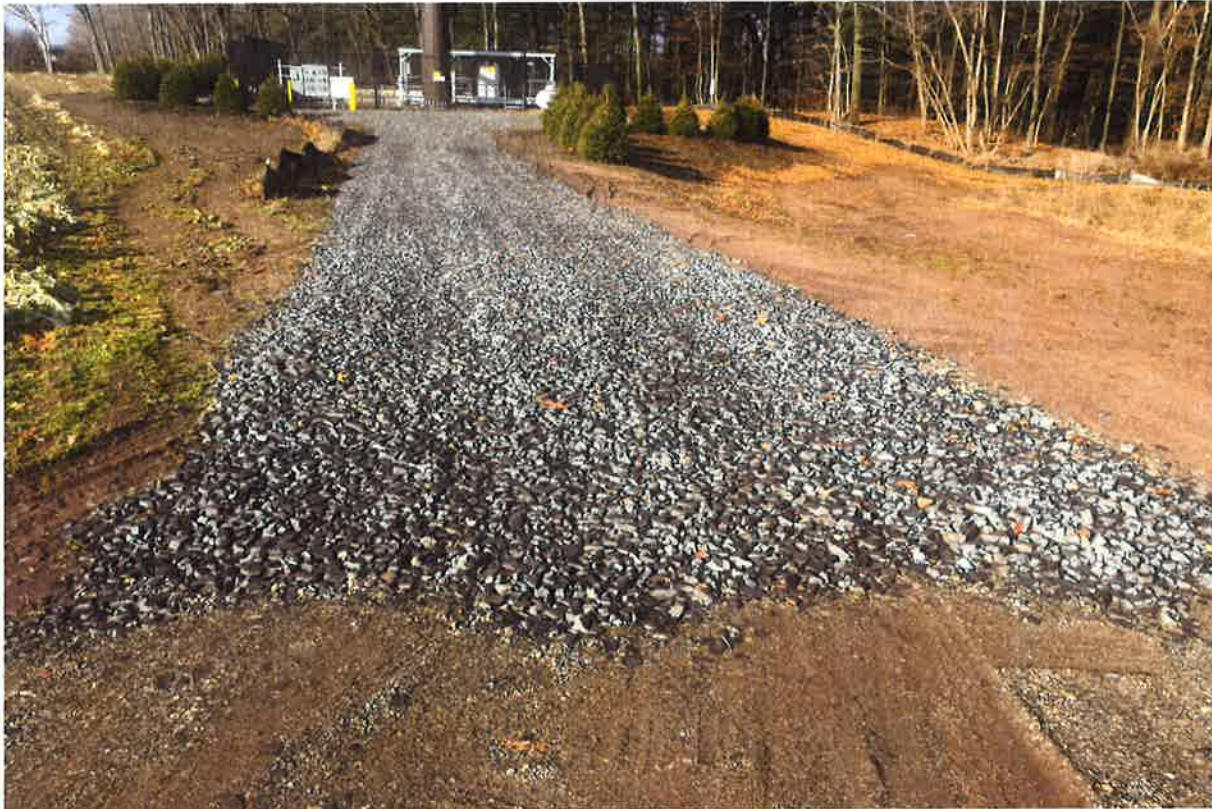
Photo 1: View of access road looking north.
