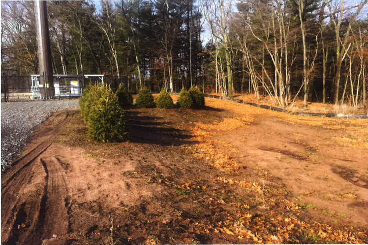
Photo 3: View of east side of compound area looking north.
