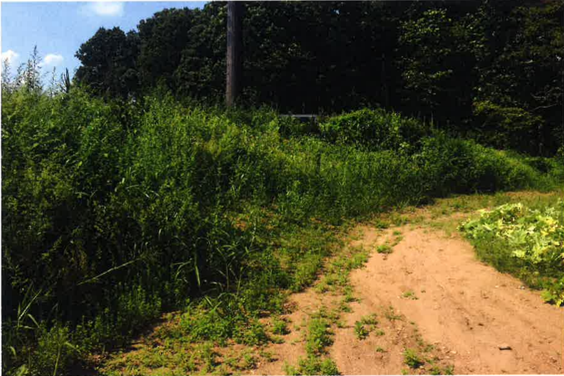
Photo 3: View of eastern side-slope looking north.
