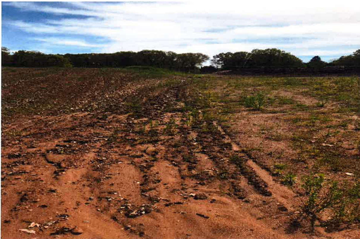
Photo 2: View of erosion patterns originating from non-Verizon related mulching activities looking south.
