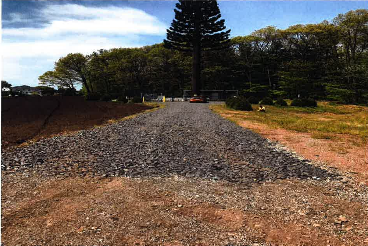
Photo 1: View of access road entrance with facility in background, looking north.
