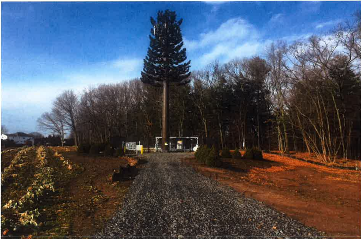
Photo 6: View of tower and compound area looking north.
