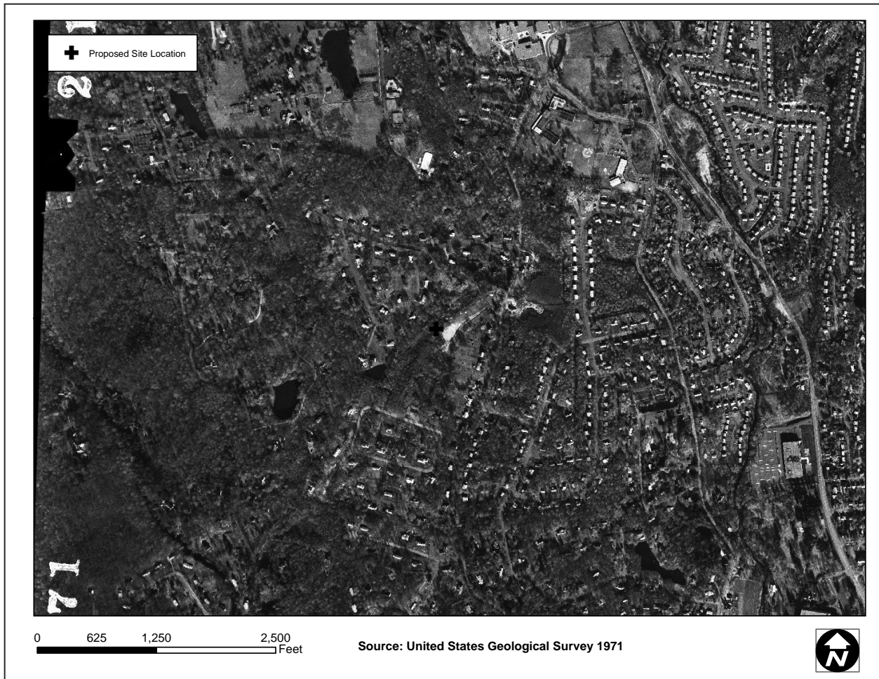
Figure 8. Excerpt from a 1971 aerial image, depicting the proposed telecommunications tower location in Stamford, Connecticut.
