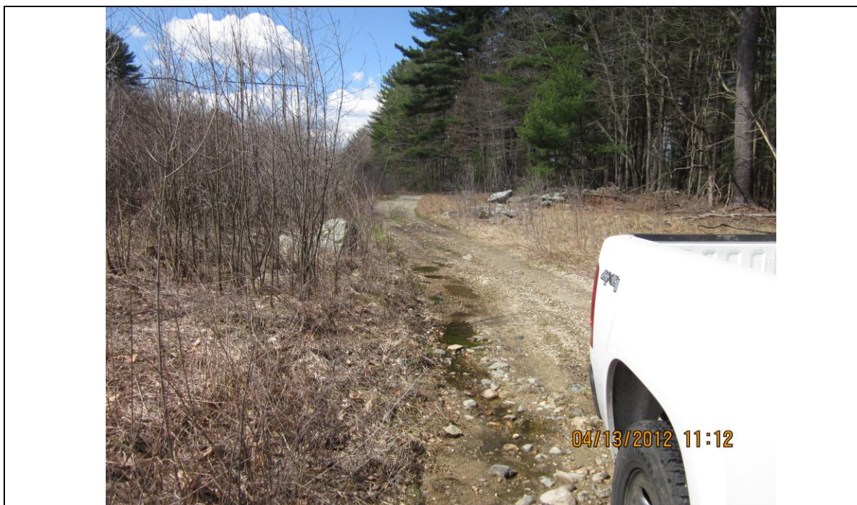
IMG_0223 Taken facing southwest on access roadway water flow entering roadway near central portion of picture. Note proposed temporary culvert is proposed for central portion of photo and water seen flowing in road infiltrates into ground before IMG_0222.
