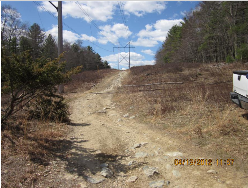
IMG_0227 Taken facing southwest at Station 1946+ showing eroded steep access road that drains towards wetlands near Rhode Island border.
