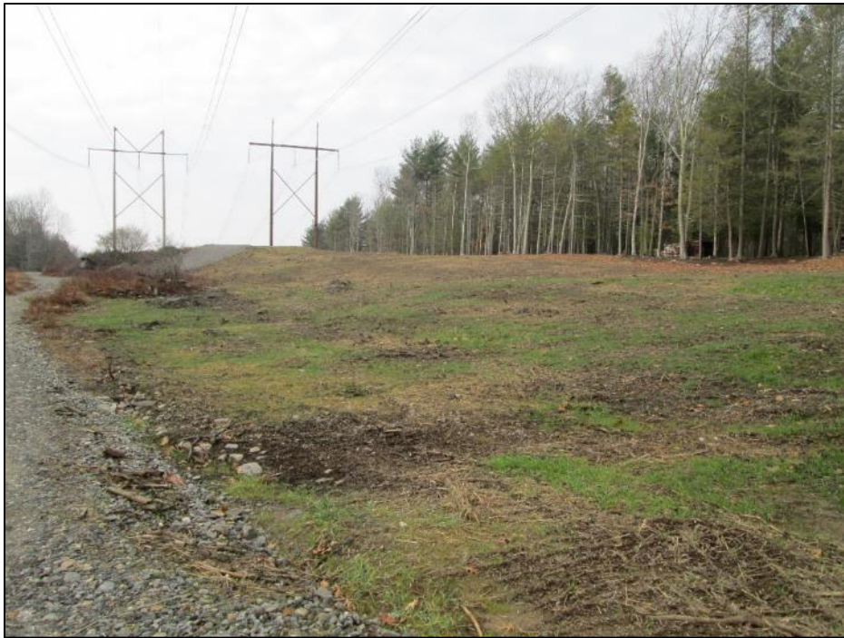
Photo #1: Str 308 not yet permanently stabilized. Typical of this area of ROW. (12/10)
