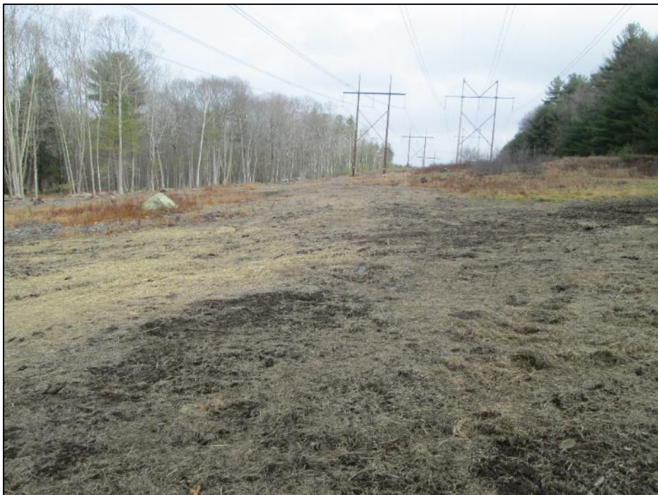
Photo #2: Str 312 not yet permanently stabilized. Typical of this area of ROW. (12/10)
