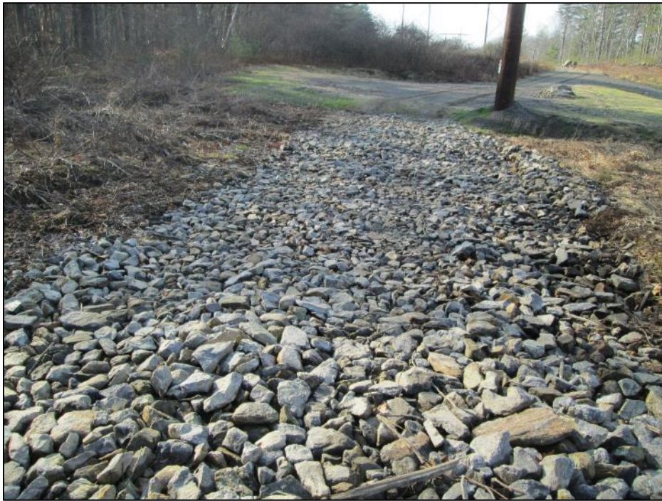
Photo #5: Rock ford to remain as permanent BMP on access road between Str 328 and 329. (12/10)
