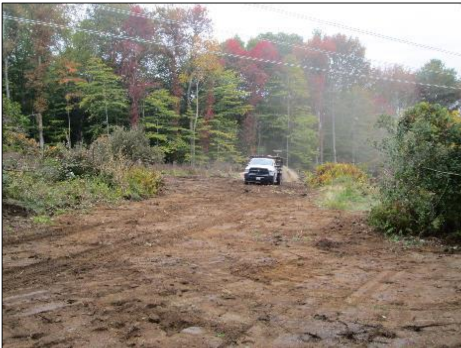
Photo #8: Blowing straw around pull pad between Str 73 and 74. (10/9)
