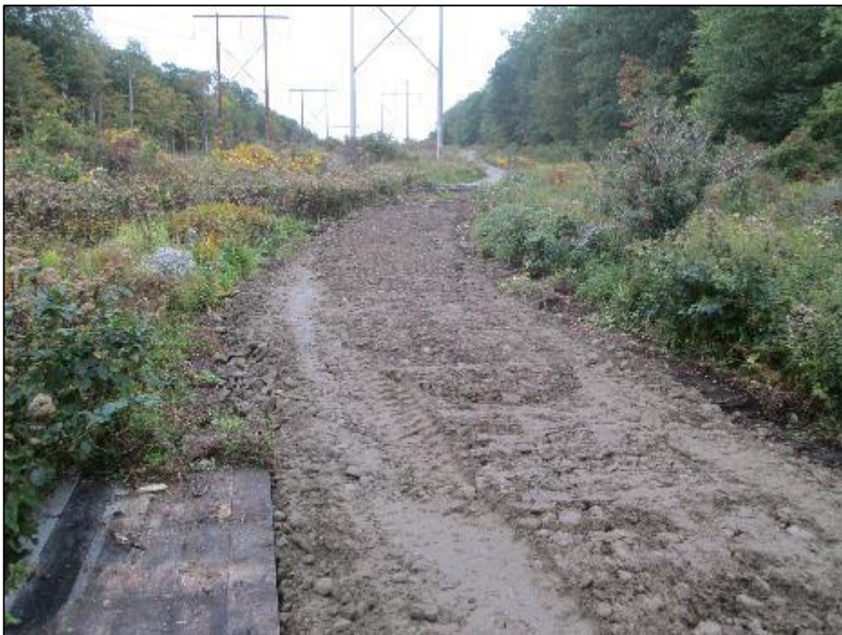
Photo #6: Str 105-106 access road being constructed as mats are removed. (10/2)
