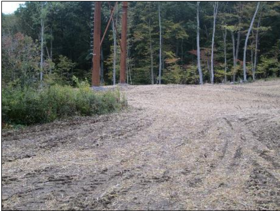
Photo #3: Str 105 seeded and temporarily stabilized with straw. (10/2)
