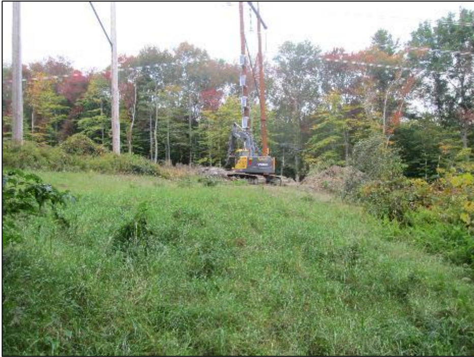
Photo #9: Earthwork and re-grading at Str 73. (10/9)
