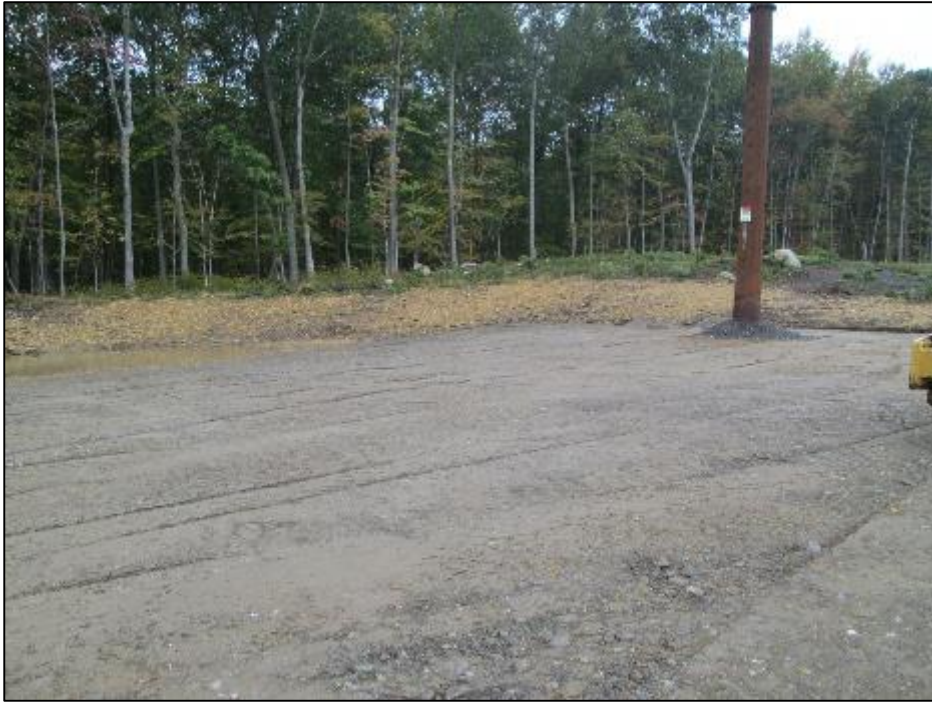
Photo #5: Restoration operations at Str 129. (10/2)
