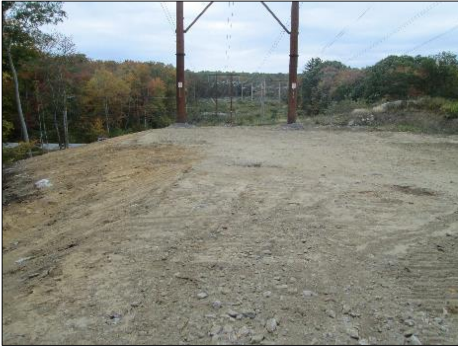
Photo #15: Site re-graded and awaiting temporary stabilization. (10/9)
