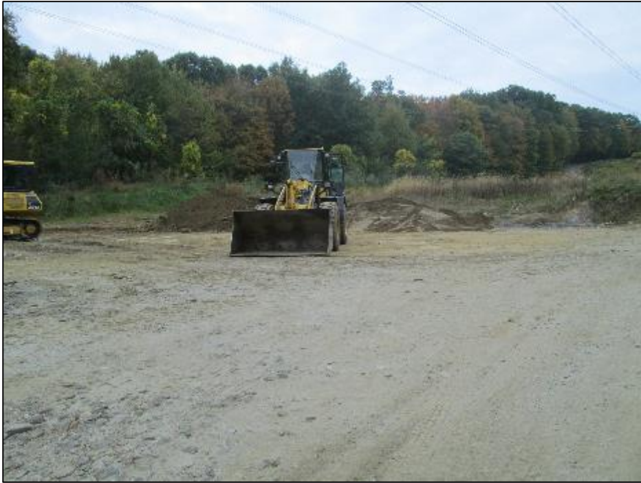
Photo #7: Earthwork and re-grading at Str 72. (10/9)
