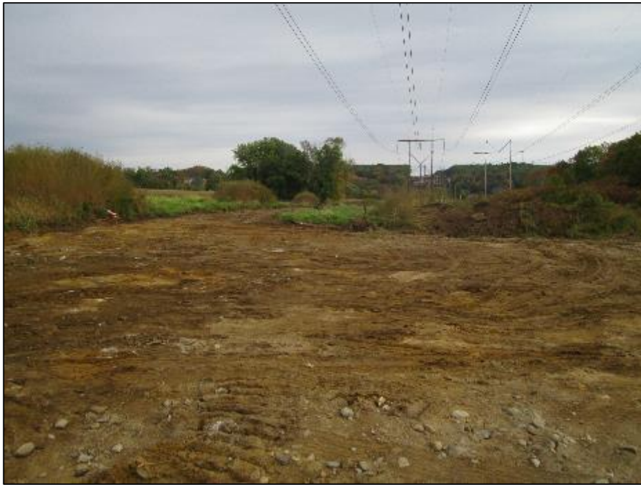
Photo #11: Construction pad removal from Str 52 area. (10/9)
