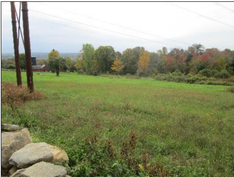
Photo #10: Final site inspection of Str 56. Site fully restored and permanently stabilized. (10/9)
