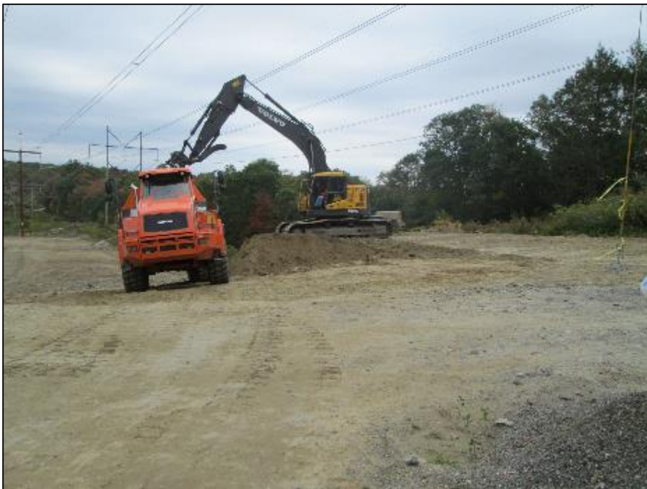
Photo #14: Removal of stone from Str 180 pad. (10/9)
